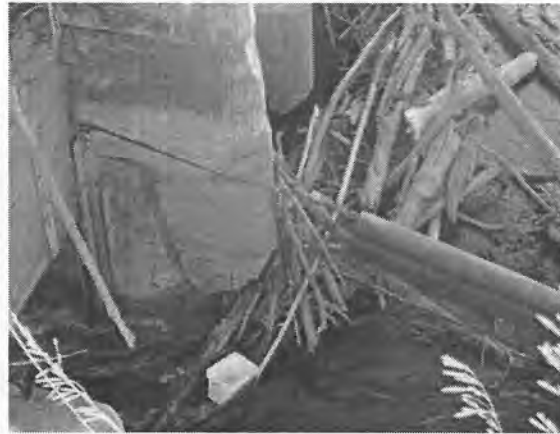
Figure 9. Concrete degradation upstream end of piers surrounding sluice bays.
