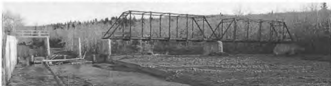
Figure 3. Existing St. Mary Dam Diversion weir, sluiceway and abandoned bridge during low flow fall season (view is from upstream left bank)
