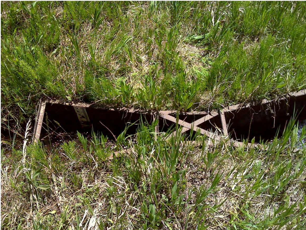
Figure 5. Photograph of 6-in. Parshall Flume on Farmers Florida Ditch diversion near the Horse Gulch siphon, N37.28947° W107.79643°.
