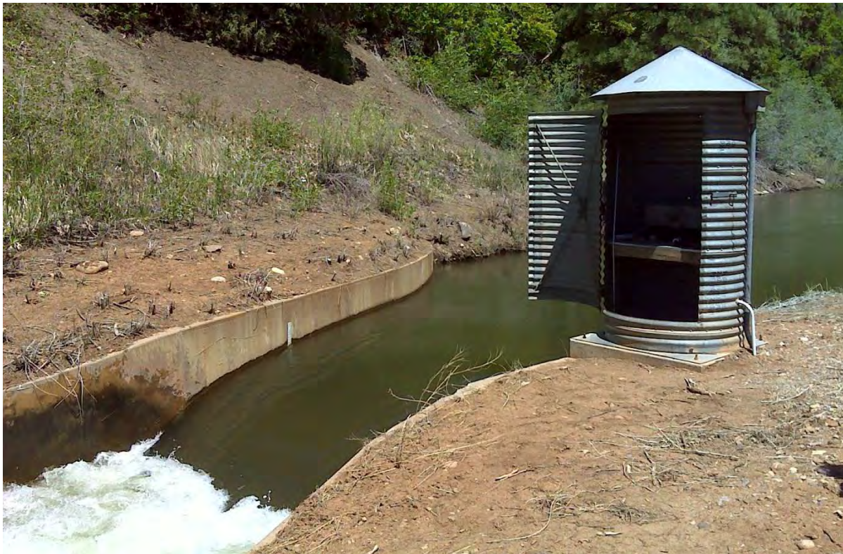
Figure 4. Photograph of 10-ft concrete Parshall Flume and water stage recorder used to monitor Florida Farmers Ditch diversions ( DWR Site: FARMERCO ).
