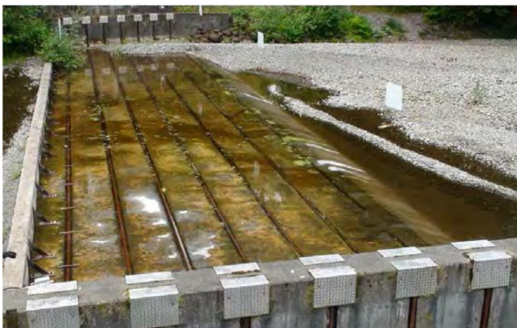
Figure 2. Example of an electric barrier with bottom flush-mounted electrodes at Quinault Fish Hatchery, Washington.
