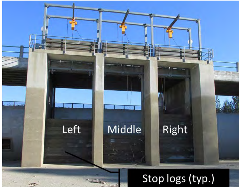
Figure 7. Photograph of Interim Flume intake in the dry (looking downstream).
