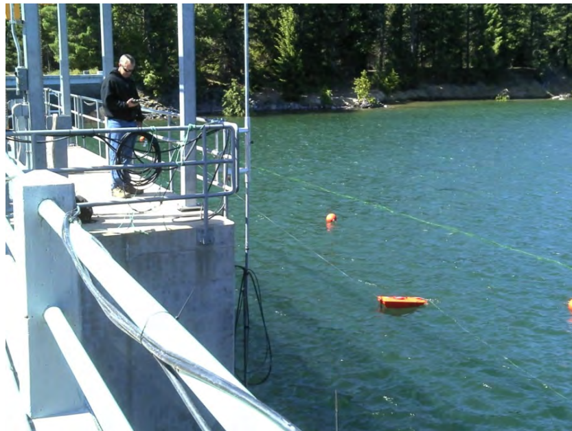
Figure 8. Photograph of tagline across forebay and QLiner float with guidance ropes. The buoys are part of a safety line across the forebay.
