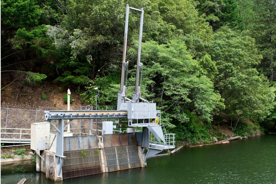
Figure 5 - Hydraulic rake (hand rake style) with support structure (image courtesy of AtlasPolar.com).
