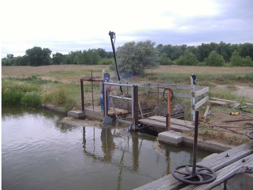
Figure 8. Newly Installed Overshoot Gate at the SPDC Spill Structure
