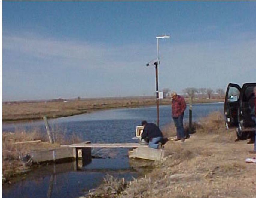
Figure 2. 2005 Installation at the SPDC Sandhill Pond Entrance
