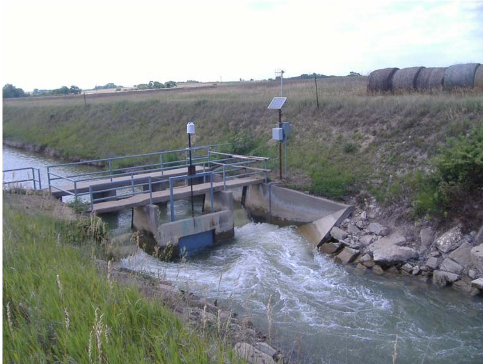
Figure 5. Completed Hardware Installation at the Nebraska Bostwick 20.2 Check
