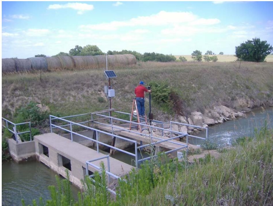
Figure 4. Reclamation Engineer Clinton Powell Making Wiring Connections on the Linear Actuator at the Nebraska Bostwick 20.2 Check
