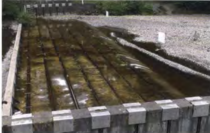
Figure 2. Main deck of concrete slab electric barrier with gravel-cobble deposition on downstream end of the southern side of Cook Creek.
