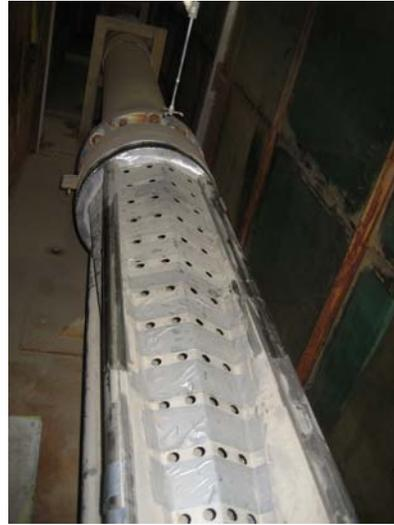
**Figure 2. Collection header – holes 75% blocked.**
