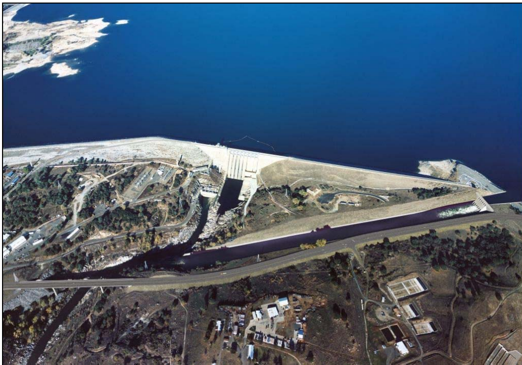
Figure 3. Artist's rendering of the new auxiliary spillway structure to the left of the main dam spillway structure. The new Folsom Lake Crossing Bridge across the American River is shown just downstream from the confluence area.
