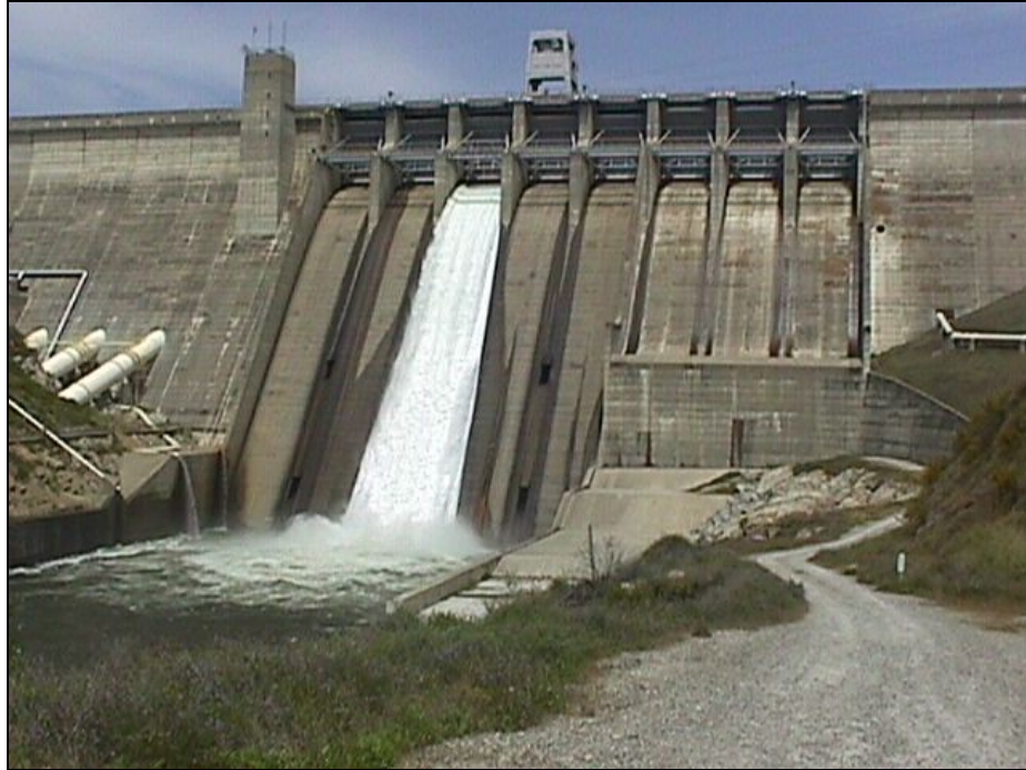
Figure 2. Concrete gravity section of Folsom Dam.
