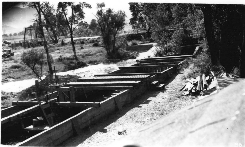
Fig. 3 Metergate and Flume Viewed from Downstream Calibration 48-in Armco Metergate Model No. 101 Colorado A & M College Hydraulics Laboratory, Bellvue, Colorado
