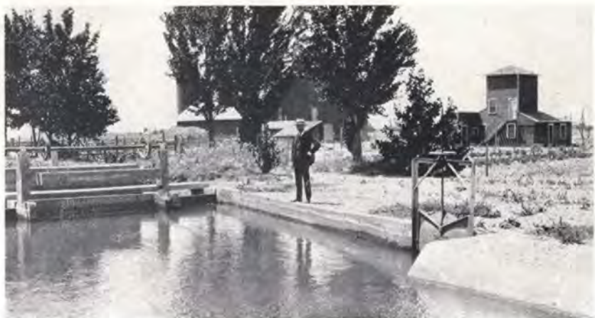
Calco Automatic Radial Gate maintaining constant level in canal. Calco Slide Headgate at right.
