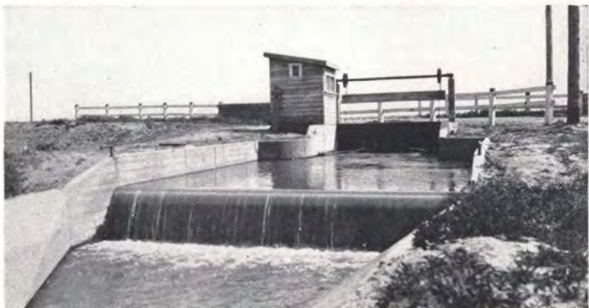
Calco Automatic Radial Gate installed to maintain constant level downstream. West Stanislaus Irrigation District, California. W. F. Woolley, Chief Engineer.
