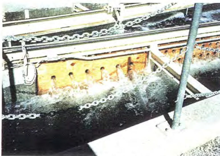
Figure 34. Temporary plywood baffles. Plywood sheets with holes cut out created temporary baffles behind the wedge-wire screens.
