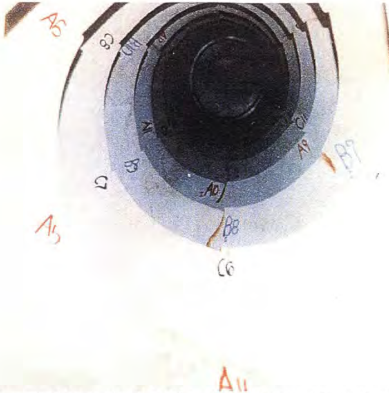
Figure 20. Cracks on the flights of Archimedes Pump 1. View looking up the barrel of Pump 1, cracking of the flights, note that crack visibility was enhanced by rust.
