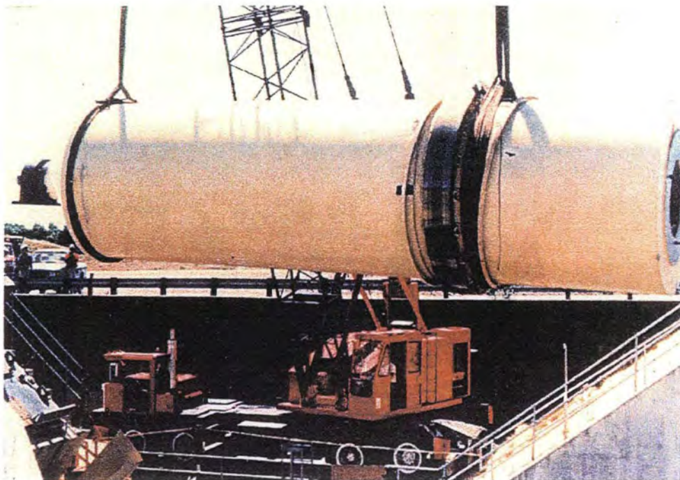
Figure 18. Removal of Pump 1 from bay. Removal of pump 1 by mobile crane in order to repair thrust bearing.
