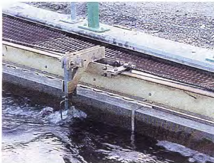
Figure 33. Sweeper in action. Continuous operating sweepers run back and forth over the wedgewire screen, brush extends the full depth of the channel.
