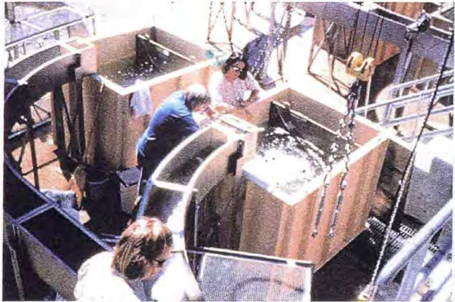
Figure 41. Holding facility. Holding tanks are able to catch the bypass flow, allowing for collection of fish which have come through the pumps.
