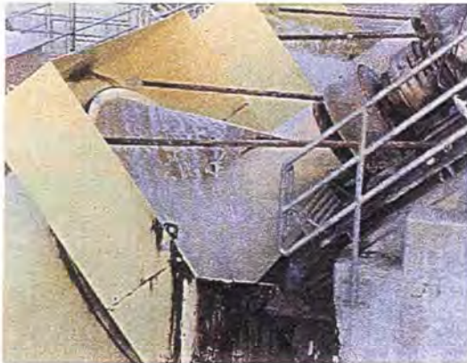
Figure 30. Archimedes pump discharge. Discharge area for the Archimedes pumps. Left photo shows the end of the pumps while the right photo shows the discharge channel after about 17 ft of channel length.
