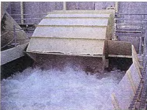
Figure 31. WEMCO-Hidrostal pump discharge. Wemco centrifugal-helical pump discharging about 80 ft 3 /s into screening channel. Left photo shows offset discharge to channel. Right photo shows channel and a portion of the vee screen structure.
