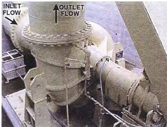
Figure 25. Flow path through the Wemco-Hidrostal Pump. This photo shows the flow direction in the Wemco-Hidrostal (36X36) pump installed at RBRPP.
