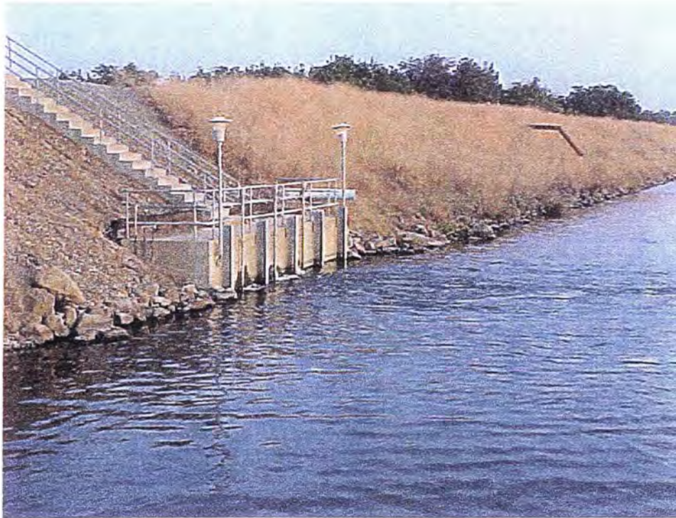
Figure 42. Terminal structure for the screened flows from RBRPP. Water flows which are screened in the vee-screen structures flow through buried pipelines and exit into the Tehama-Colusa canal at the structure shown above. Propeller-type flowmeters measure the flow from each pipe flowing into the canal.
