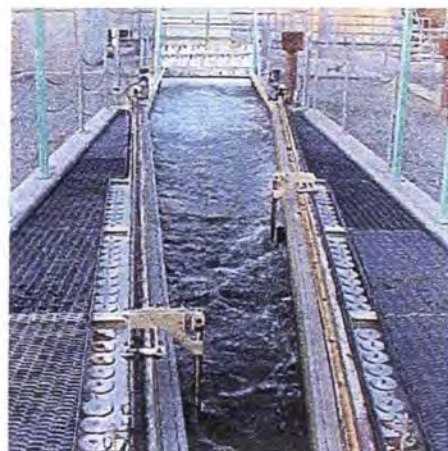
Figure 31. WEMCO-Hidrostal pump discharge. Wemco centrifugal-helical pump discharging about 80 ft 3 /s into screening channel. Left photo shows offset discharge to channel. Right photo shows channel and a portion of the vee screen structure.
