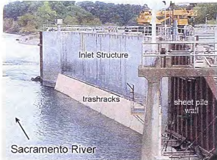
Figure 9. Inlet structure including trashracks. The inlet structure to the RBRPP includes 160 ft of trashracks with 45-degree angled bars with 2\frac{1}{2} inch openings.
