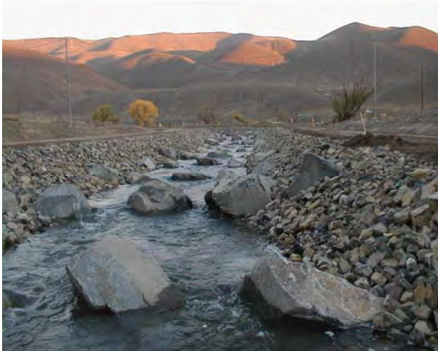
Figure 6- View of the Derby Diversion Dam roughened-channel fishway, Truckee River, NV.
