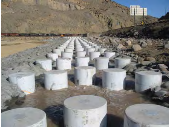
Figure 7 – Looking upstream at the cylinder baffles in the Price-Stubb Dam roughened-channel fishway, Colorado River, Co.
