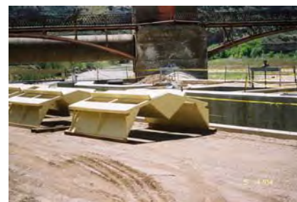
Steel baffles prior to installation in the fishway.
