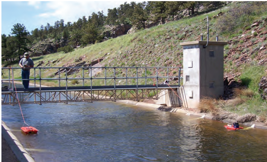
Figure 1: Gauging station on the Hansen Feeder Canal where section-by-section measurements were made. Teledyne/RDI StreamPro on the right side, OTT QLiner on the left side, deployed from the current metering bridge.
