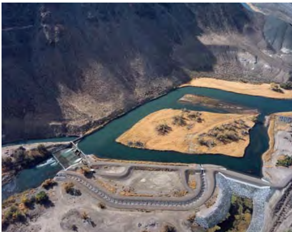
Figure 7 - Photographs of Derby Diversion Dam rock channel and boulder weir fishway.
