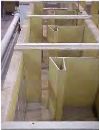
View of standard vertical slot baffle fishway looking downstream.
