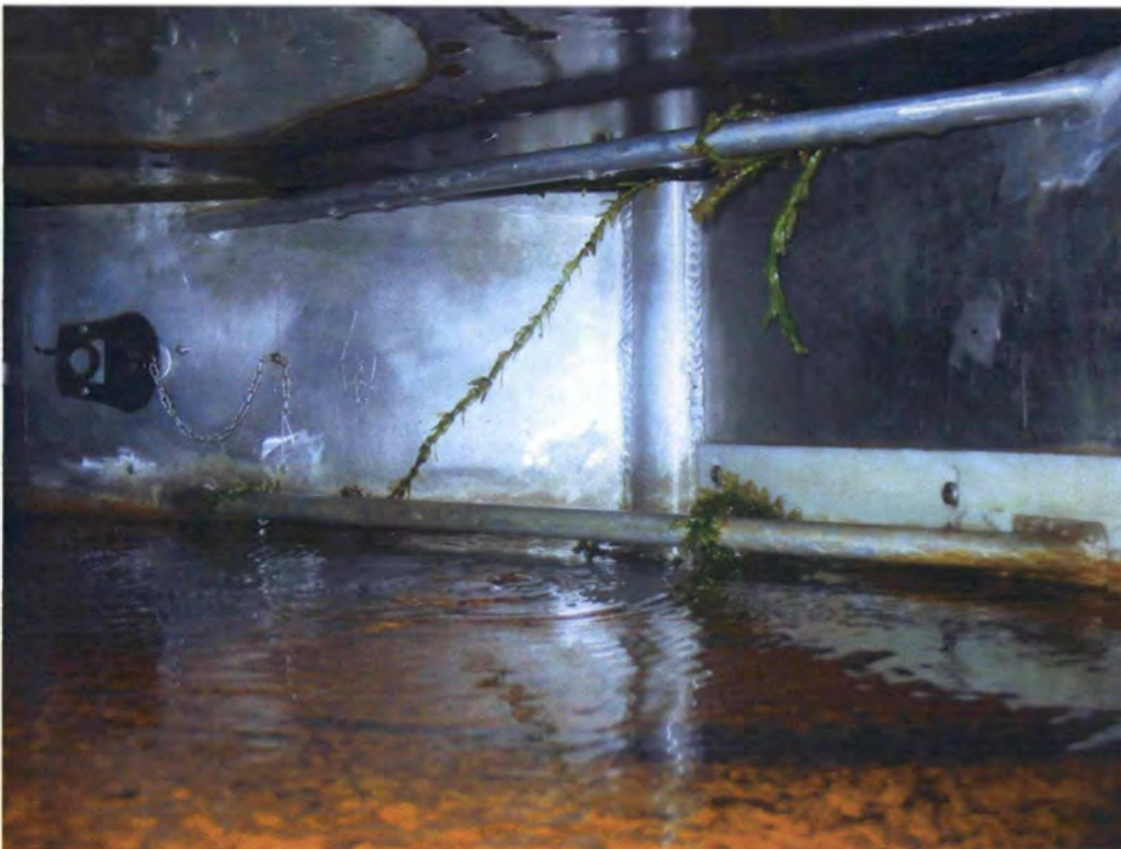
Figure 18– View looking at center of rotary vane. Note pond weed on vane support struts.
