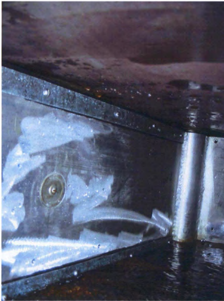
Photograph 2– View of vane with support bars removed. Also note metal strips holding rubber flaps at the vane edges.
