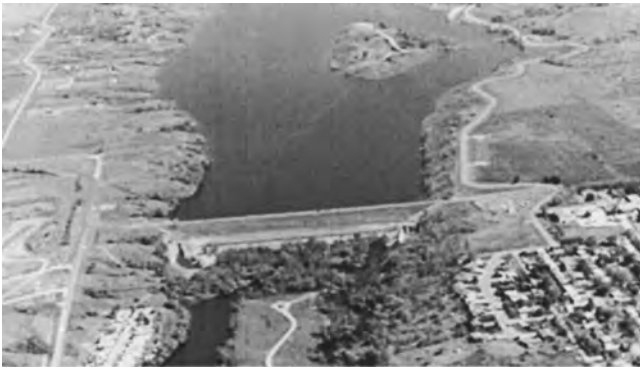
Fig. 2. Aerial photo of the dam and reservoir considered in the case study application
