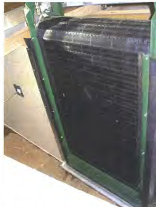
Figure 2. - Traveling screen installed in the WRRL recirculating flow facility. The screen shown in the right photo is mounted vertically on a 10 degree converging wall between the two walkways spanning the facility.
