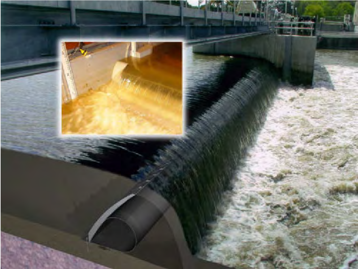
Figure 11. Obermeyer Gate.
