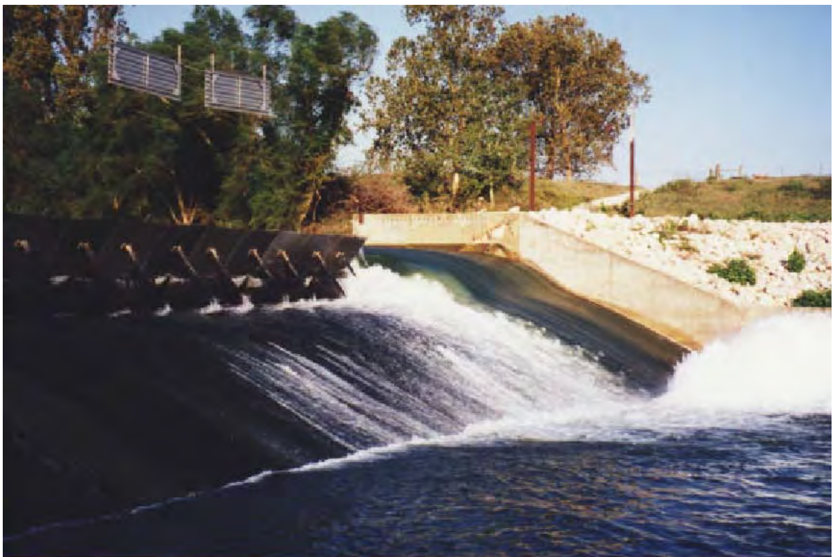
Figure 13. Obermeyer Gates on a concrete crest. Note independent operation of gate sections.
