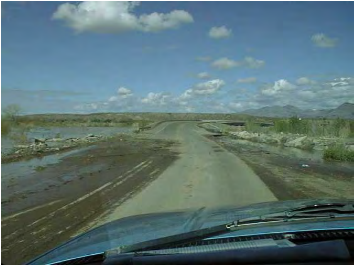
Figure 7. Left abutment and approach to Solomon Bridge. Note that the approach has recently been inundated (flow right to left) by floodwaters.
