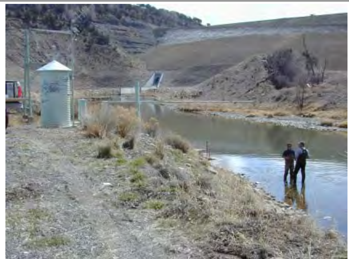
Figure 9. - The USGS river gage station about 750 ft downstream from the dam. Note the walls of the spillway stilling basin can be seen in the background. Also notice the shallow water at this site. This is typical of the small bypass releases that occur.
