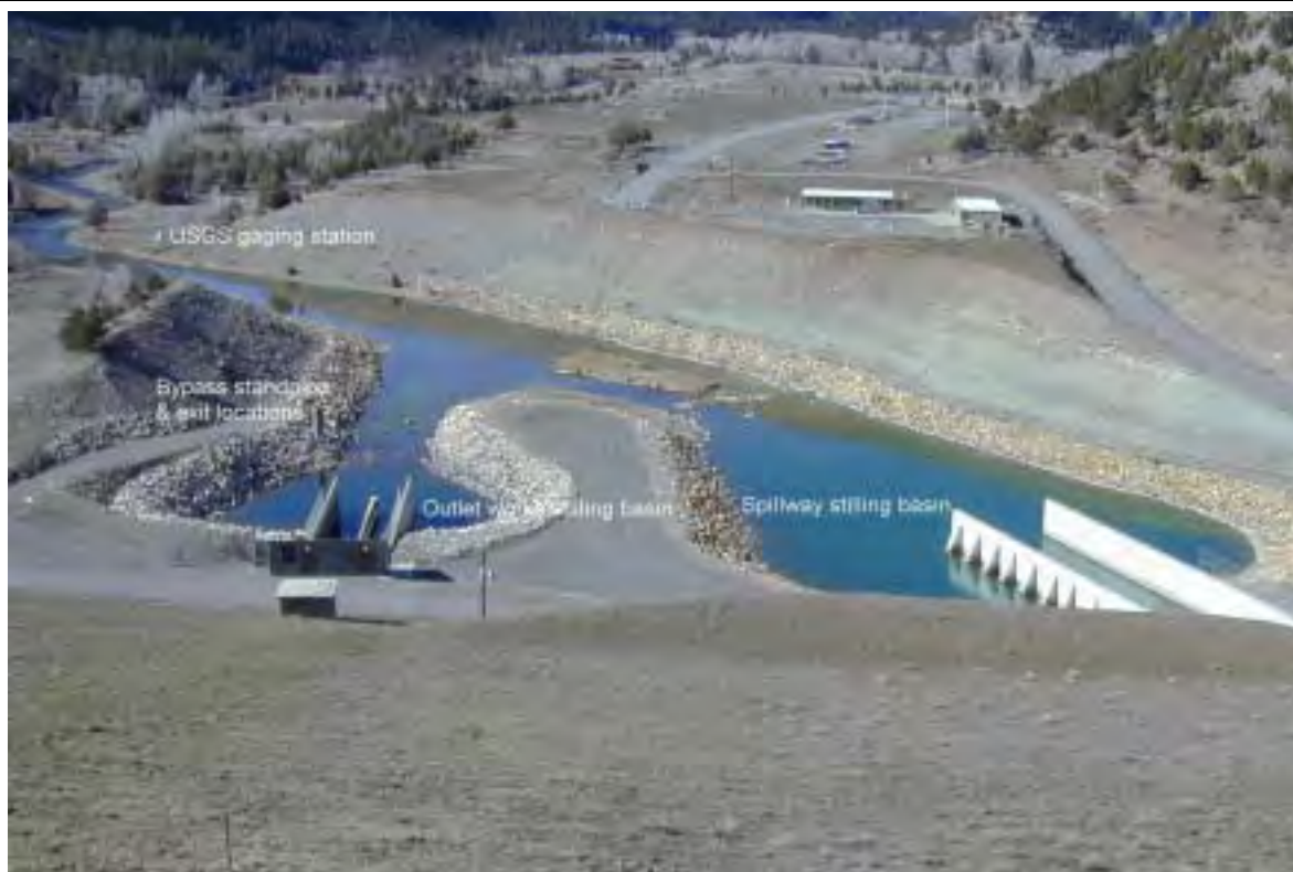
Figure 1. – Downstream view of Ridgway Dam outlet works and spillway stilling basins and a short section of the river. The bypass pipe has been relocated into the left side of the narrow channel just downstream from the outlet works stilling basin.
