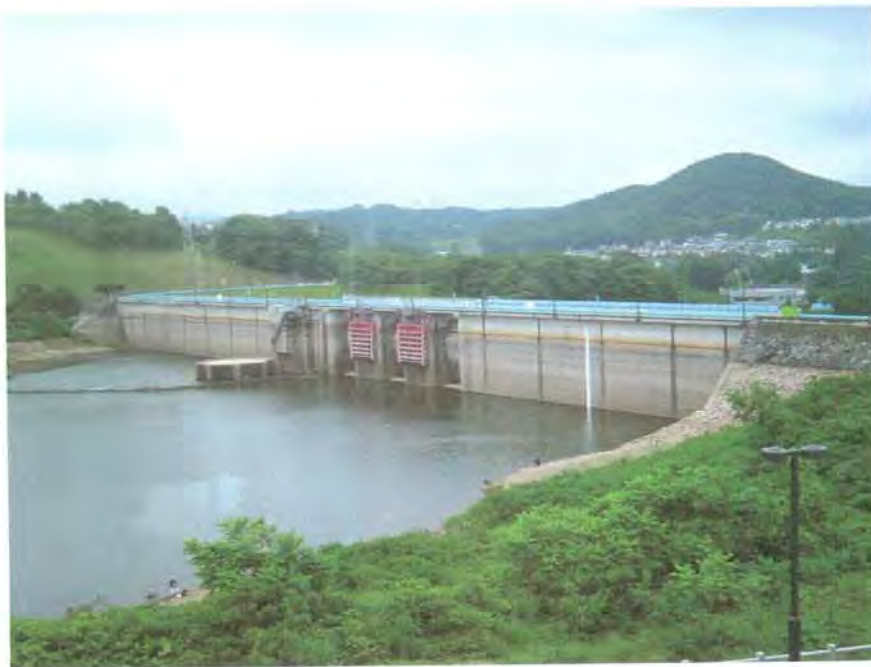
Shijushida Dam, Iwate, July 19, 2003
