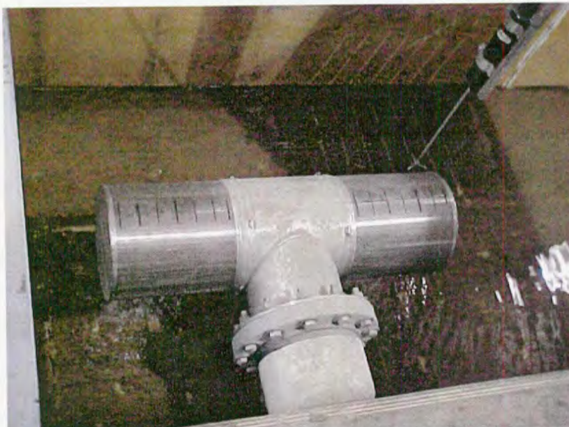
Figure 1. Hendrick 12 inch tee screen.
