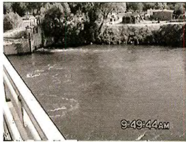
View of surface flow conditions downstream of the left bank fishway.
