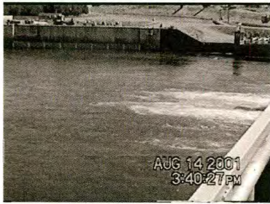
View of white water turbulence downstream of gates 5, 6 and 7.
