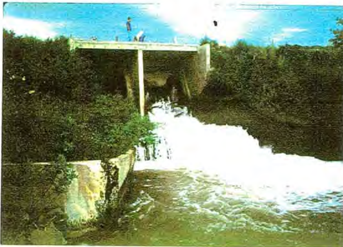
Figure 7 - View looking upstream at the Burns Wasteway flow control gates.
