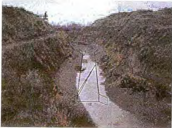
Figure 6 - View looking upstream toward the Main canal headworks. Photo was taken from the access bridge to the Intake boat launch and recreation area. Outline of the screen structure shows the approximate location.
