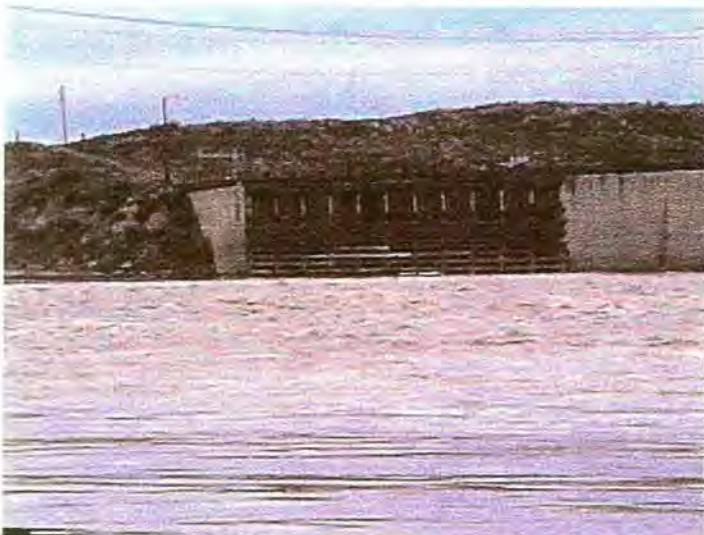
Figure 2 - View of Intake Dam and Main Canal Headworks.
