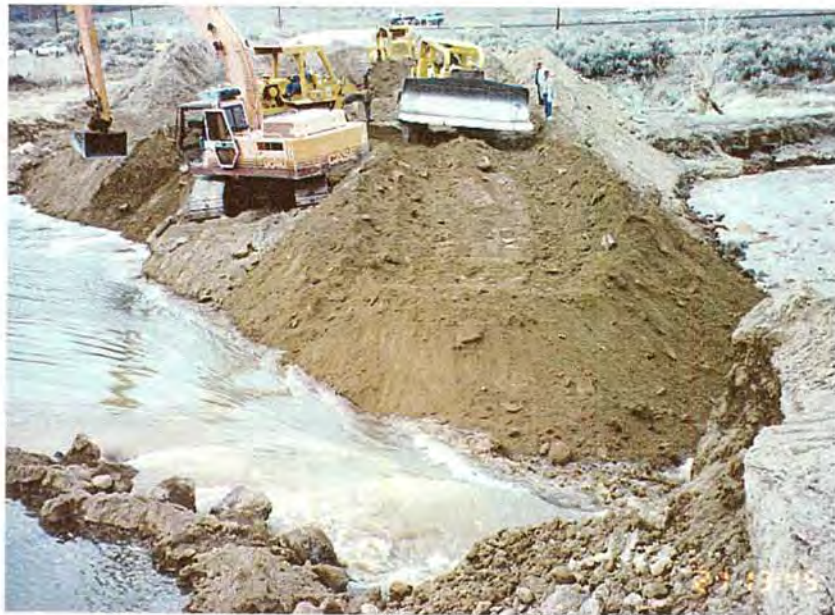
Figure 23 - Replacement of the soft plug following 1997 breach.
