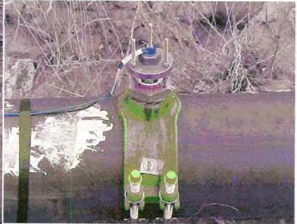
Figure 7. - Data Industrial paddle wheel flow rate sensor installed on an 8 in pipeline. These meters may be used on pipes between 3 and 26 inches in diameter.
