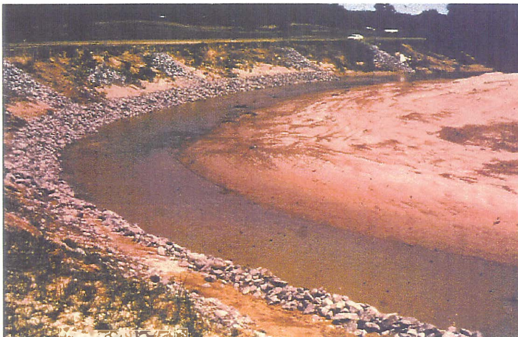
Figure 5. Typical longitudinal peaked stone toe protection with tie-backs (from Biedenbarn, Elliot, & Watson. 1998)
