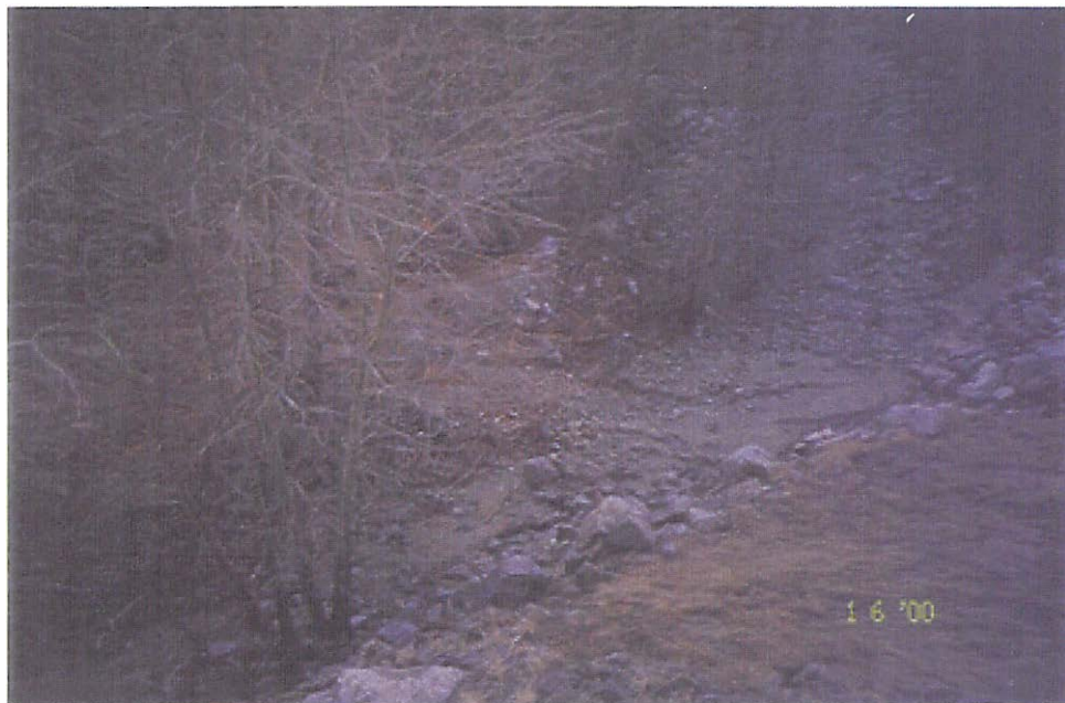
Photograph 0898-69. Left bank longitudinal peaked stone toe protection in Bend #26.
