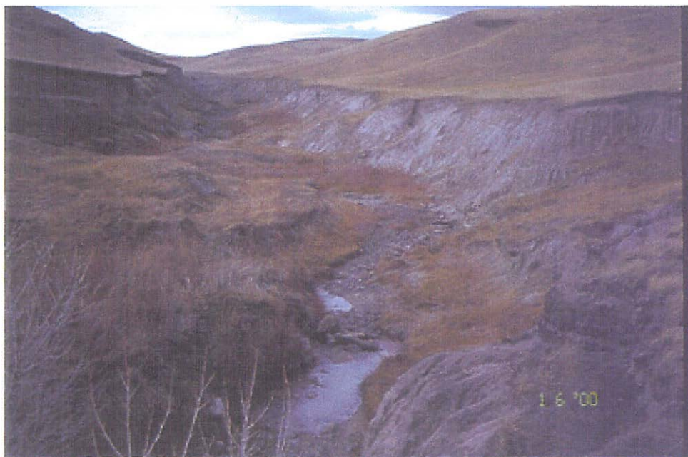
Photograph 0898-24 (54+60). Both banks looking US at Bend #12 and Straight Reach #5. Note view upstream showing potential access along left bank for construction equipment. Low probability that those vehicles could traverse upper left bank. Access in channel adequate for tracked vehicles only.
