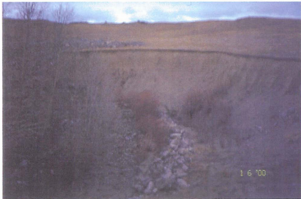
Photograph 0898-71. Left bank and riparian area created behind longitudinal peaked stone toe protection. Panned up from Photograph 0898-70.
