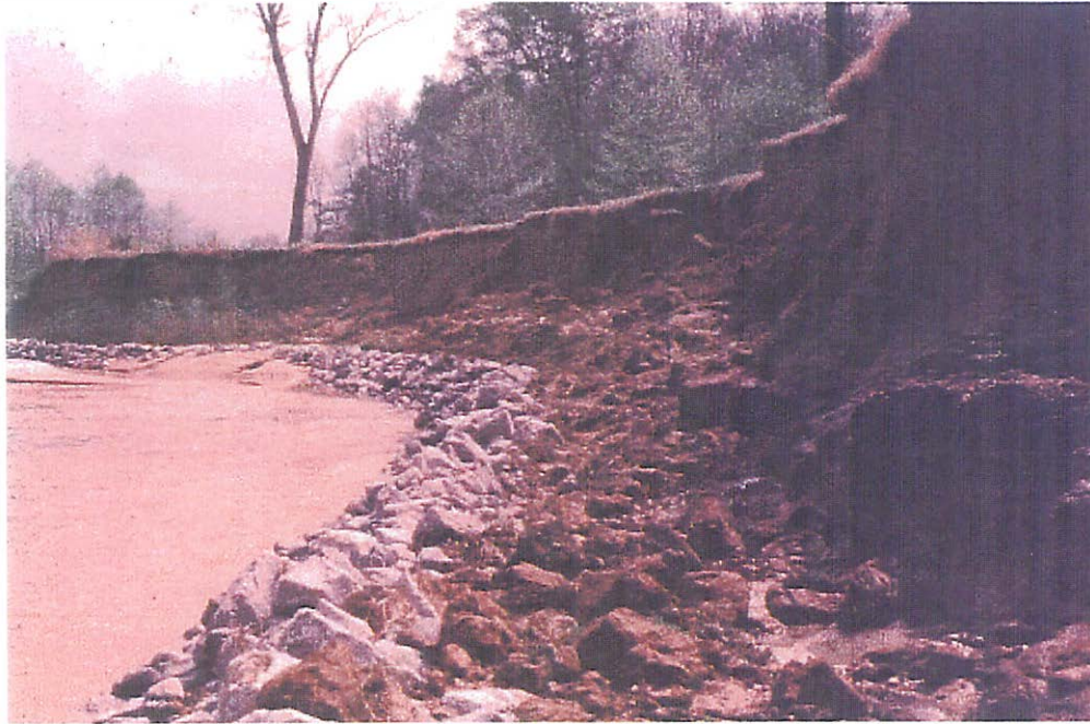
Figure 4. One ton per foot immediately after construction. (from Biedenbarn, Elliot, & Watson. 1998)
