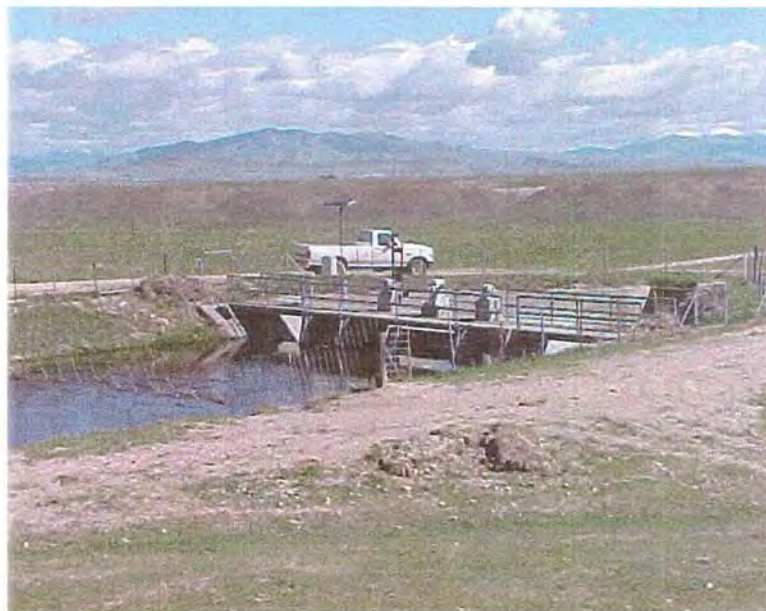
Figure 8 - Check Structure on East Bench Canal
