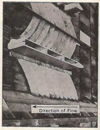
FIG. 4.--- A RIFFLE-DEFLECTOR, VORTEX-TUBE SAND TRAP
