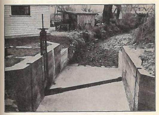
FIG. 2.---VORTEX-TUBE SAND TRAP IN JACKSON DITCH, BELLVUE HYDRAULIC LABORATORY, BELLVUE, COLO.
