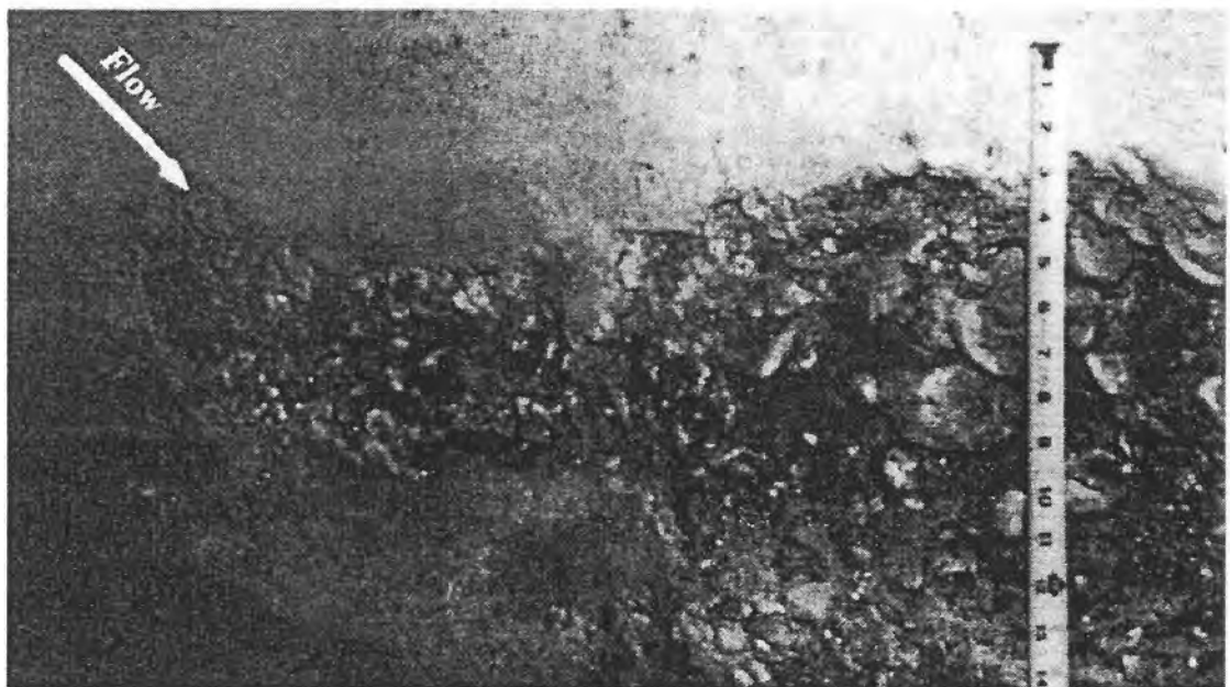
b. Hoover Dam, Nevada spillway tunnel — initiation of damage
