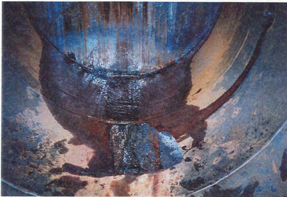
Photograph 2 - Interior view of damage to outlet pipe No. 2.
