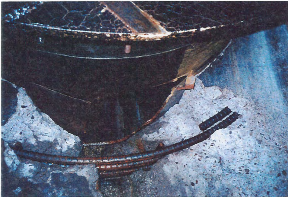
Photograph 1 - Exterior view of damage to outlet pipe No. 2.
