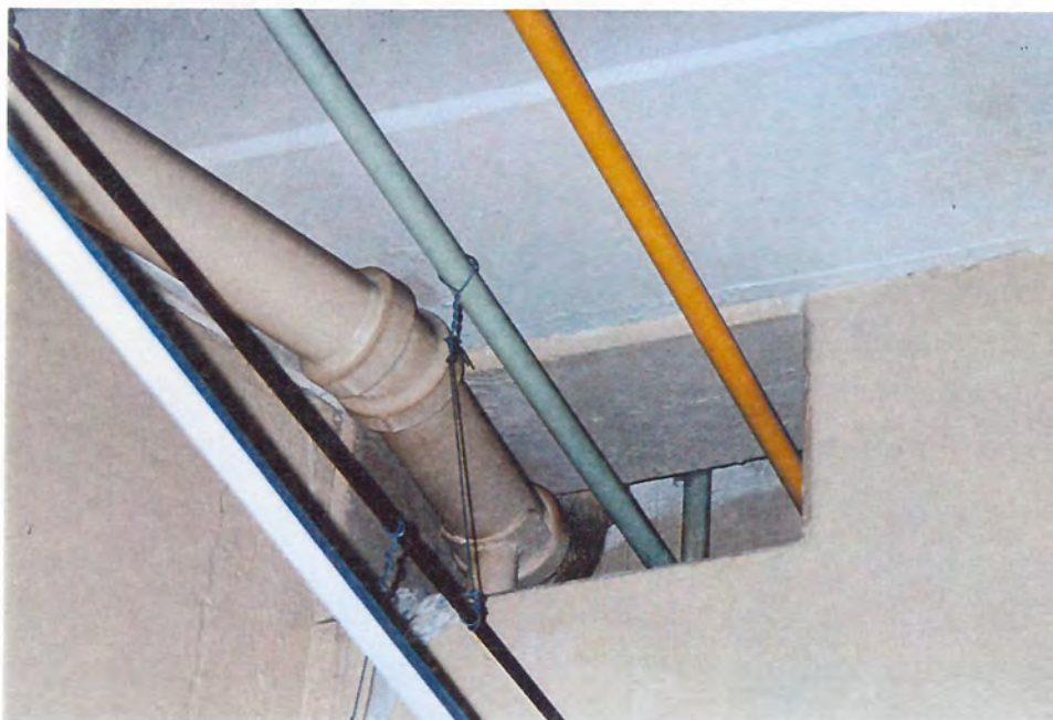
Photograph 20 - Pipe chase located between the powerplant and the control house through which water entered the powerplant.
