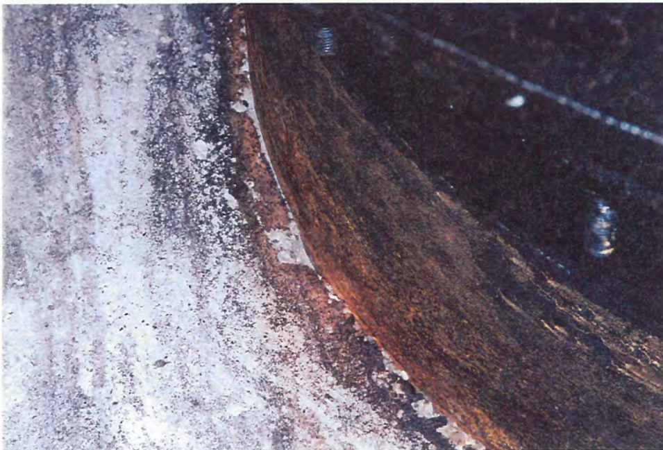
Photograph 4 - Concrete-steel outlet pipe interface. Note spalled concrete around circumference of outlet pipe which is indicative of damage caused by vibration.
