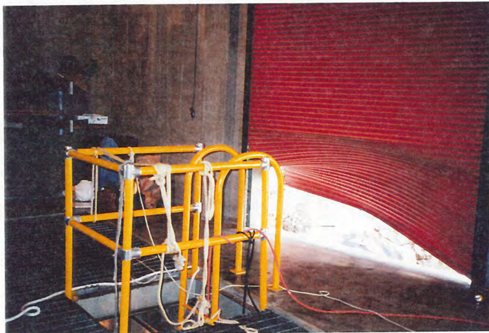
Photograph 18 - Interior view of damage to roll-up door located inside the ring follower gate control house.
