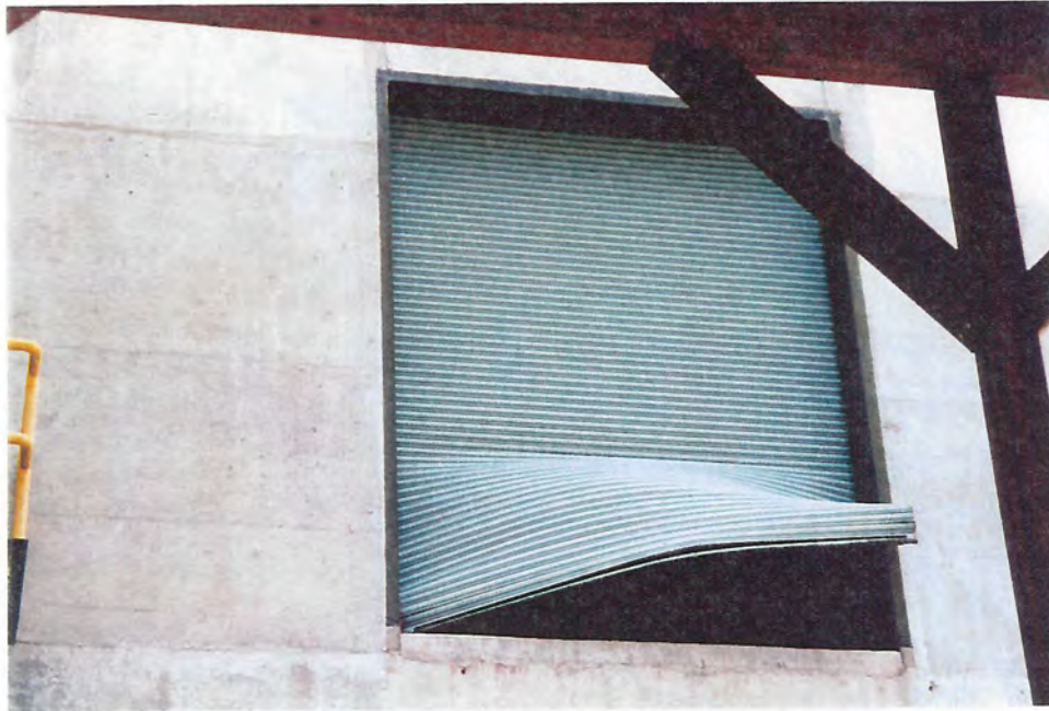
Photograph 17 - Exterior view of damage to roll-up door located in the ring follower gate control house.
