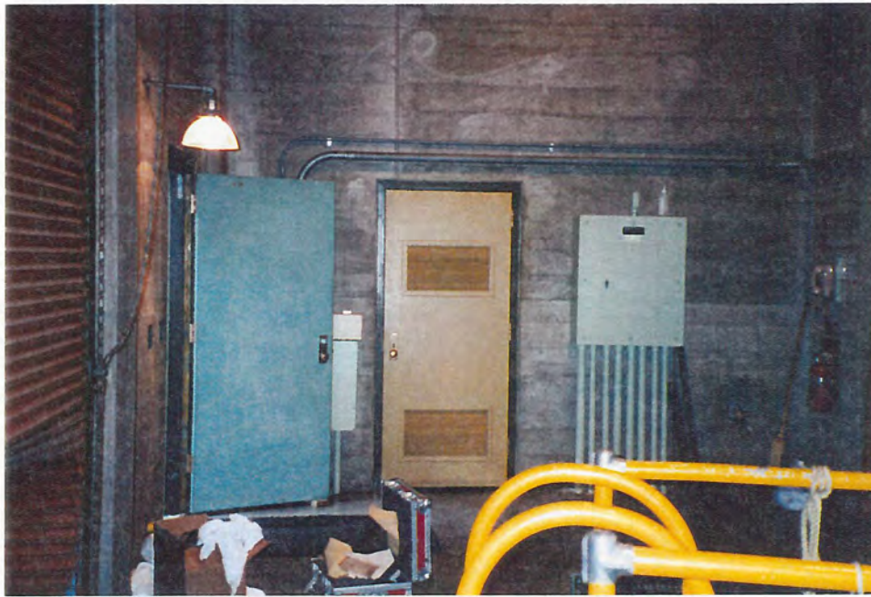
Photograph 21 - Access door between the powerplant and the ring follower gate control house through which water entered the powerplant.
