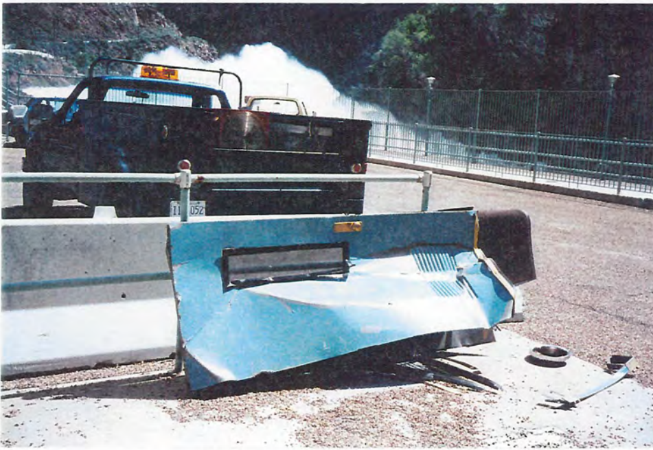
Photograph 23 - Damage to break room access door caused by flooding.
