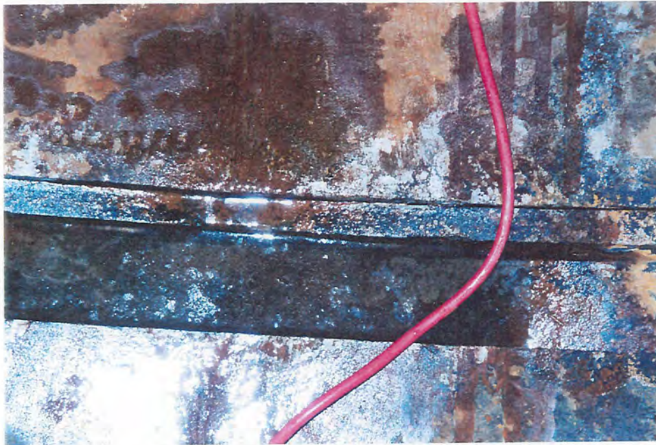
Photograph 15 - Interior view of expansion joint on outlet pipe No. 2. Note how metal stop is directly against the downstream inner sleeve.
