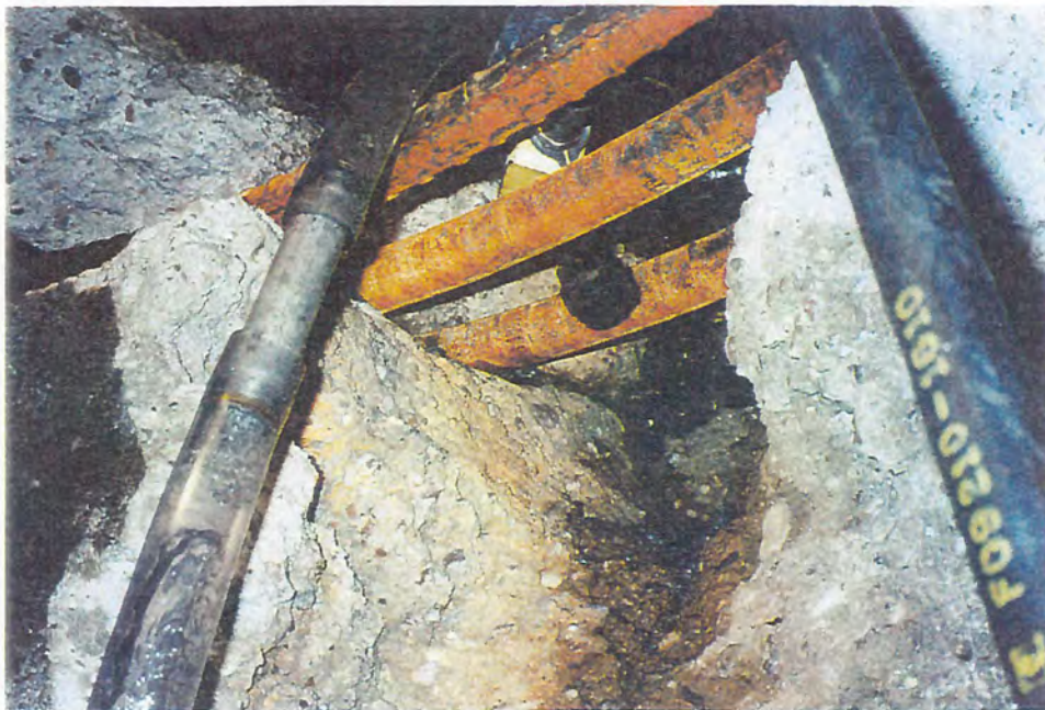
Photograph No. 5. - Showing damaged concrete and rust on reinforcement.
