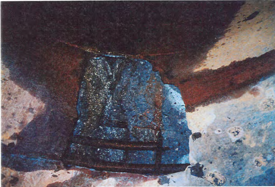
Photograph 3 - Interior view of damaged area of outlet pie No. 2.
