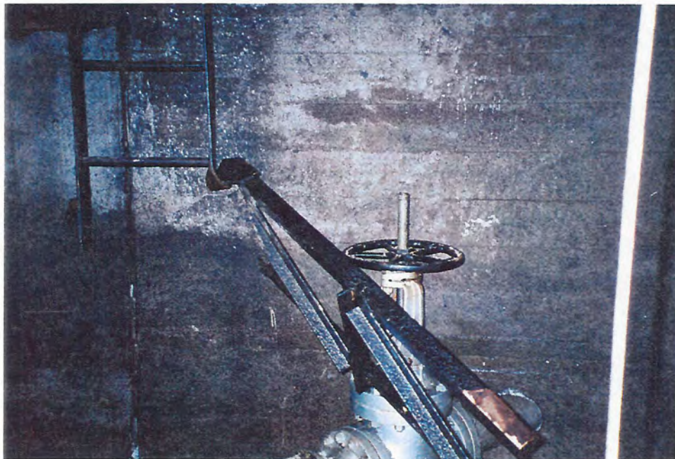
Photograph 14 - Damage caused by leakage through broken outlet pipe to access ladder which was attached to the expansion joint.
