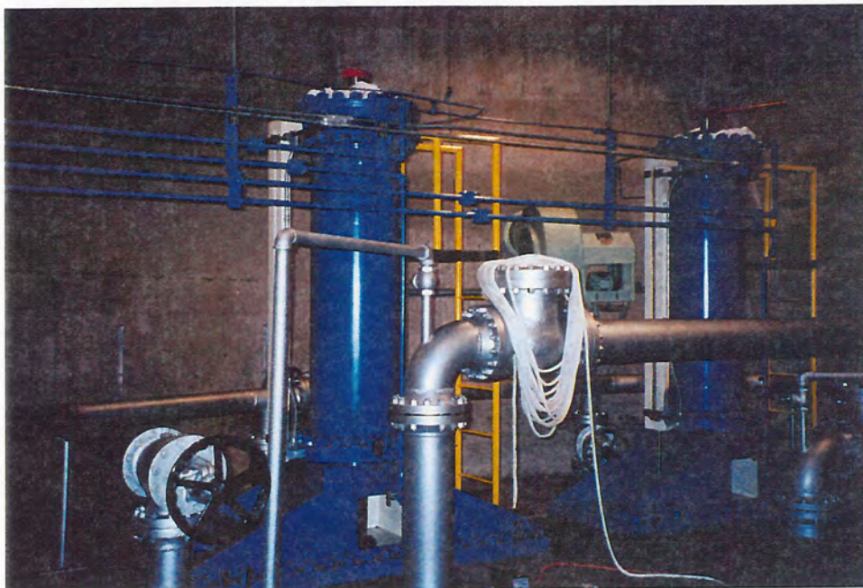
Photograph 11 - Hoist cylinders for ring follower gates located in gate control house.
