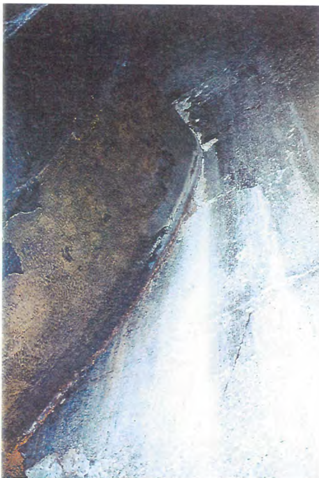
Photograph No. 3. - Note spalling around the outlet pipe.
