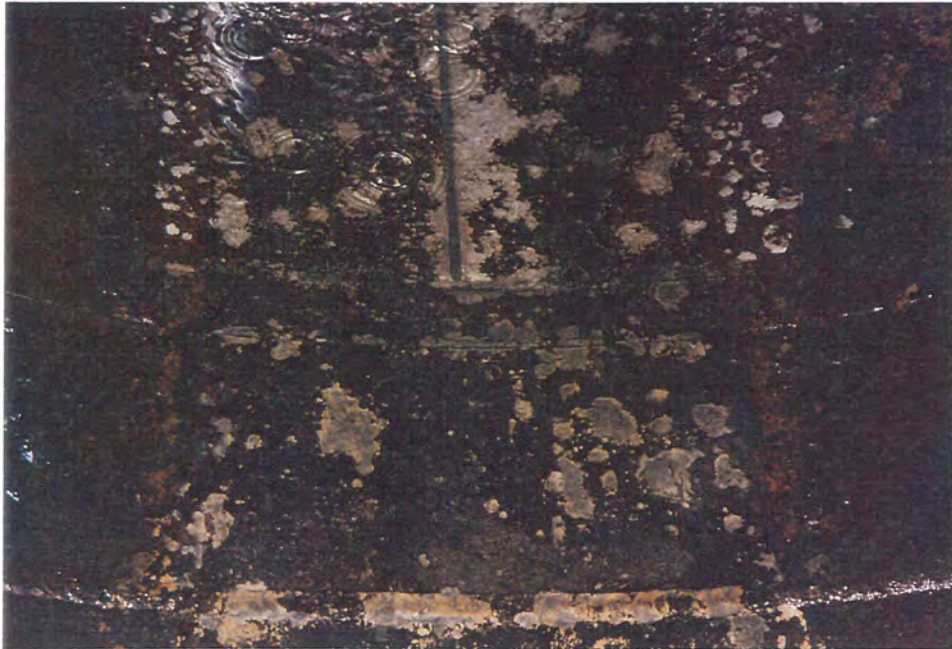
Photograph 25 - Invert of outlet pipe No. 1. Note missing coal tar epoxy but no evidence of metal loss due to cavitation.
