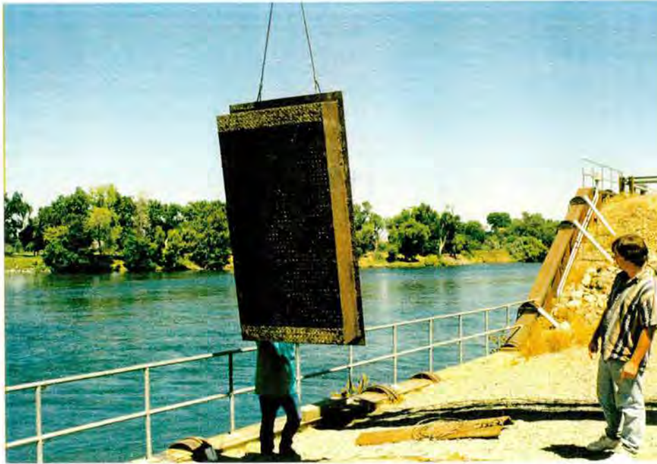
Figure 3. Photograph of orifice plug. Installed to return ladder entrance to original (pre modified) condition.
