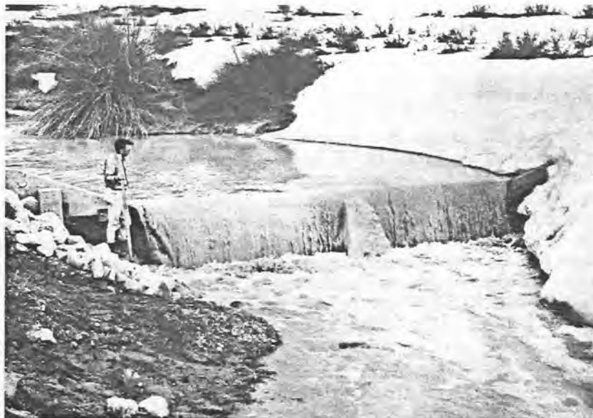
Figure 10.—This prefabricated, prestressed concrete check dam accumulated sediment readily because the structure is not porous. At the same time, dynamic and hydrostatic forces of the flow on the dam are much stronger than those at a porous rock check dam. The discharge over the spillway of this structure, installed on the Alkali Creek watershed, is about 0.4 \text{ m}^3/\text{s} .
