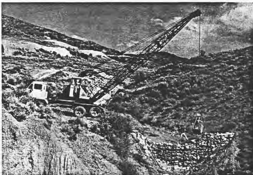
Figure 28.—Using clamshell to place rock into a double-fence dam. The man steadies the clamshell with a long rope.
