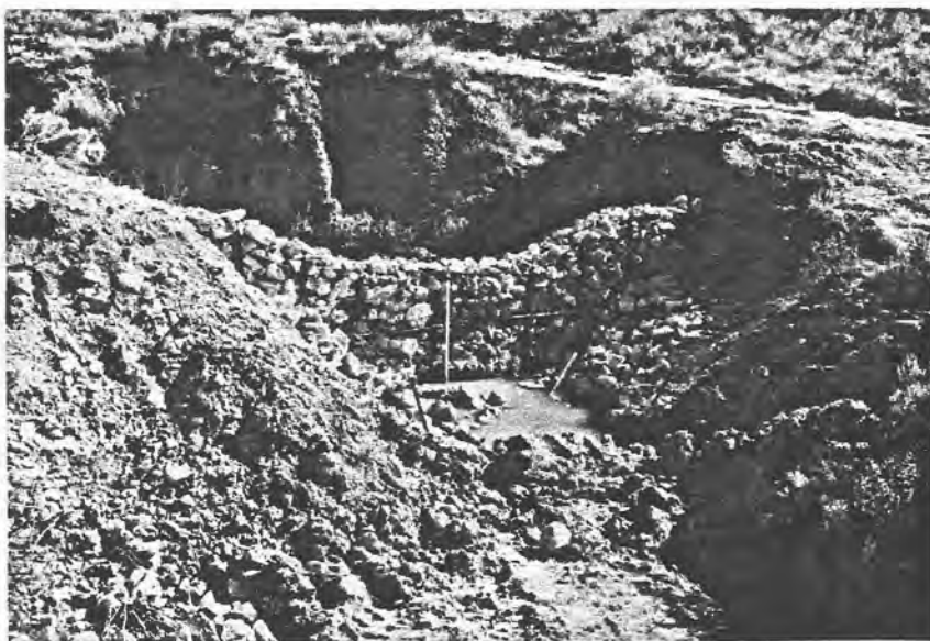
Figure 17.—Upstream view of a double-fence dam. Note the bank protection work. The apron is covered by water. Length of rod is 1.7 m.
