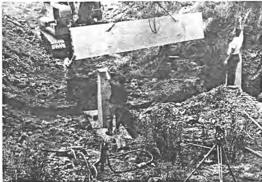
Figure 32.—Placement of a pre-stressed concrete slab against the buttresses of a prefabricated dam on Alkali Creek watershed. Backhoe proved to be sufficient for excavation of key and for structural installation. View is downstream.
