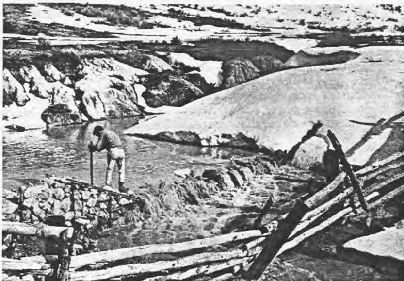
Figure 11.—As contrasted to impervious dams, rock check dams such as this double-fence structure release much of the flow, and hence hydrostatic pressure, through the structure.
