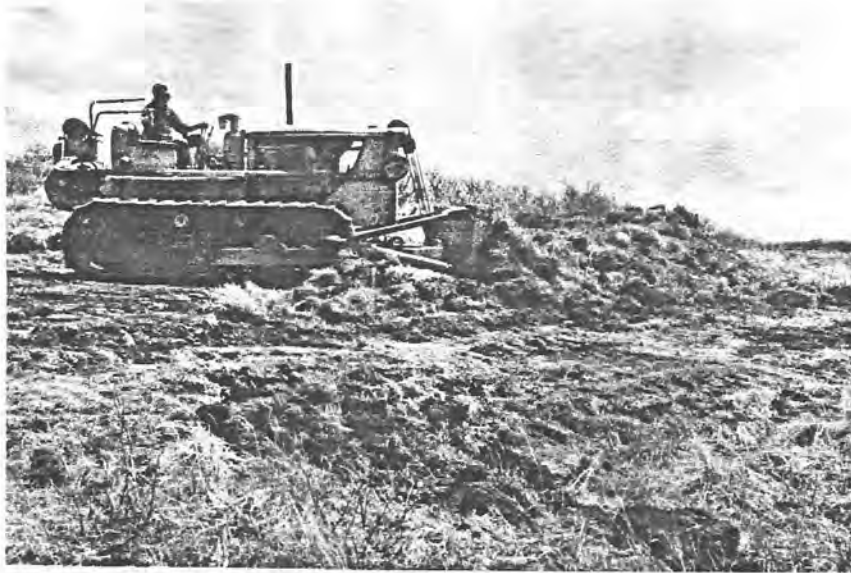
Figure 35.—Topsoil is removed from the construction area and saved, to be spread later on the finished waterway.
