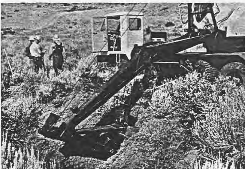
Figure 25.—The key for a rock check dam is efficiently excavated with a backhoe.
