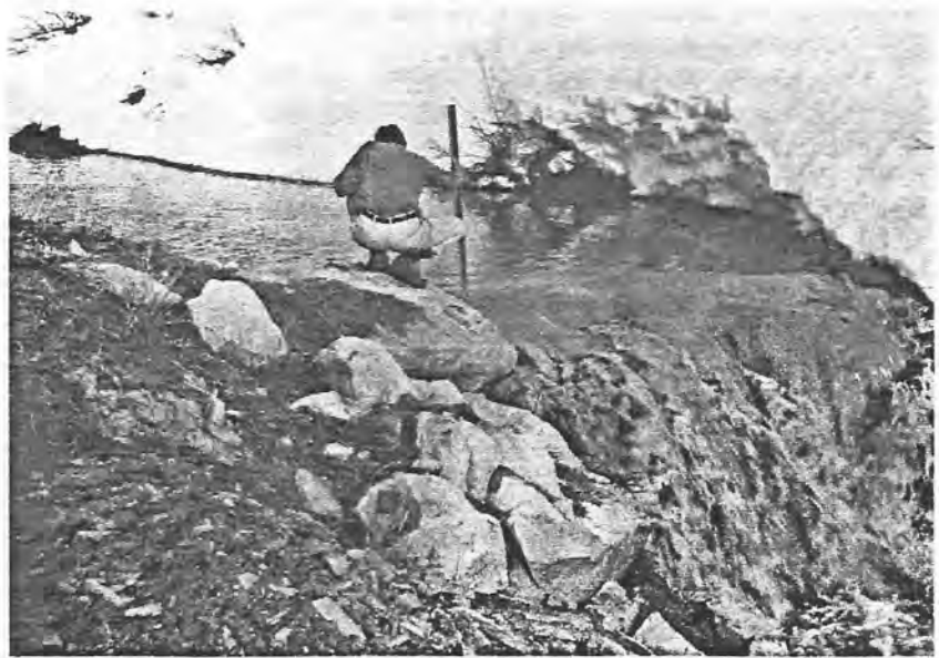
Figure 23.—Upstream view of a loose-rock check dam supporting a discharge of about 0.3 m 3 /s. Effective dam height is 1.7 m.
