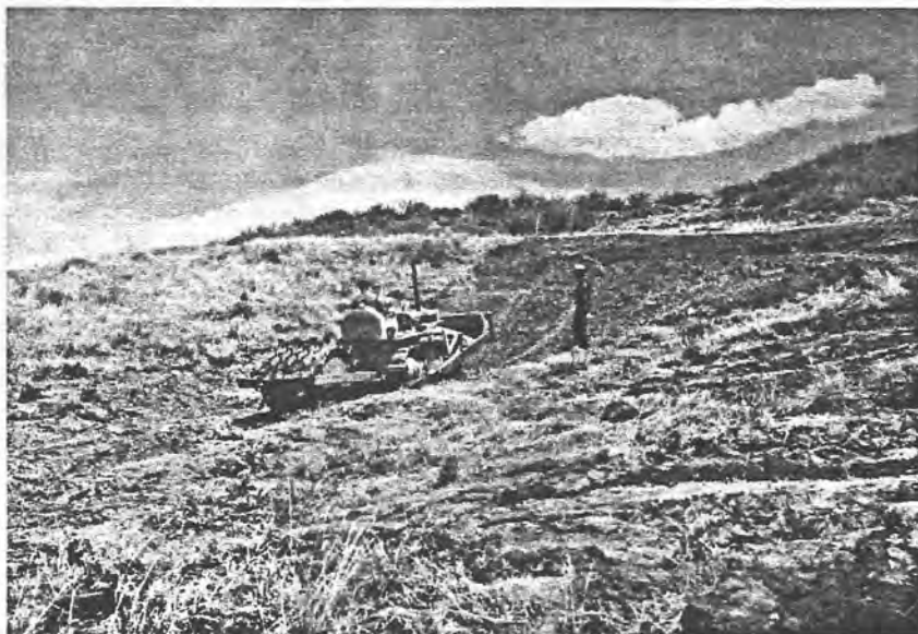
Figure 36.—A sheep-foot roller pulled by a small tractor compacts the fill in the gully. Fill was placed in layers 0.15 to 0.30 m thick.
