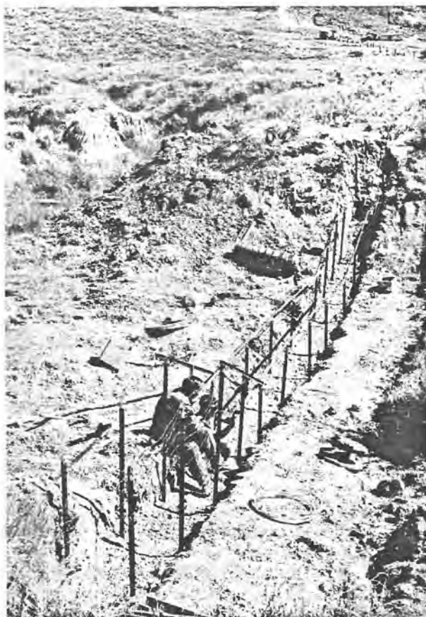
Figure 27.—Parallel fences for double-fence dam (see fig. 11) are being installed. Note the excavations for key, apron, and bank protection (the latter two to right of the structure).
