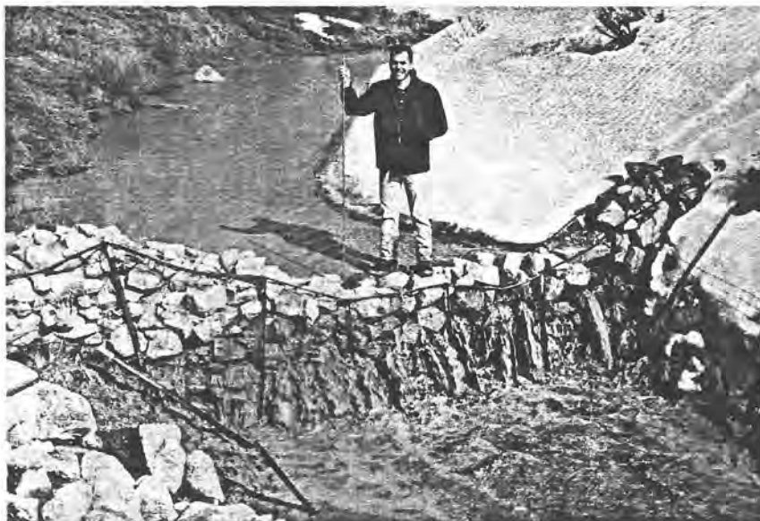
Figure 19.—Because this double-fence rock check dam was built with an insufficient portion of small rocks, many large voids allow water jets through the structure. Note that water is not running over the spillway. The jets endanger the stability of the structural keys and bank protection work.
