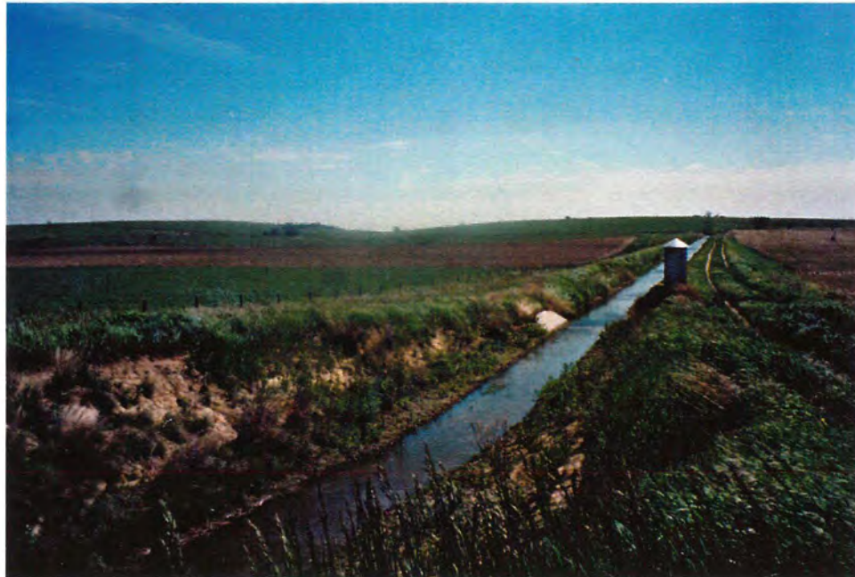
Photo 4 - Upstream segment of Lateral 6.1, with ramp flume and stilling well shelter
