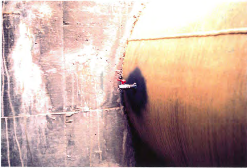
Figure 9: Piezometer tap installation on the intake pipe leading to the pumps.
