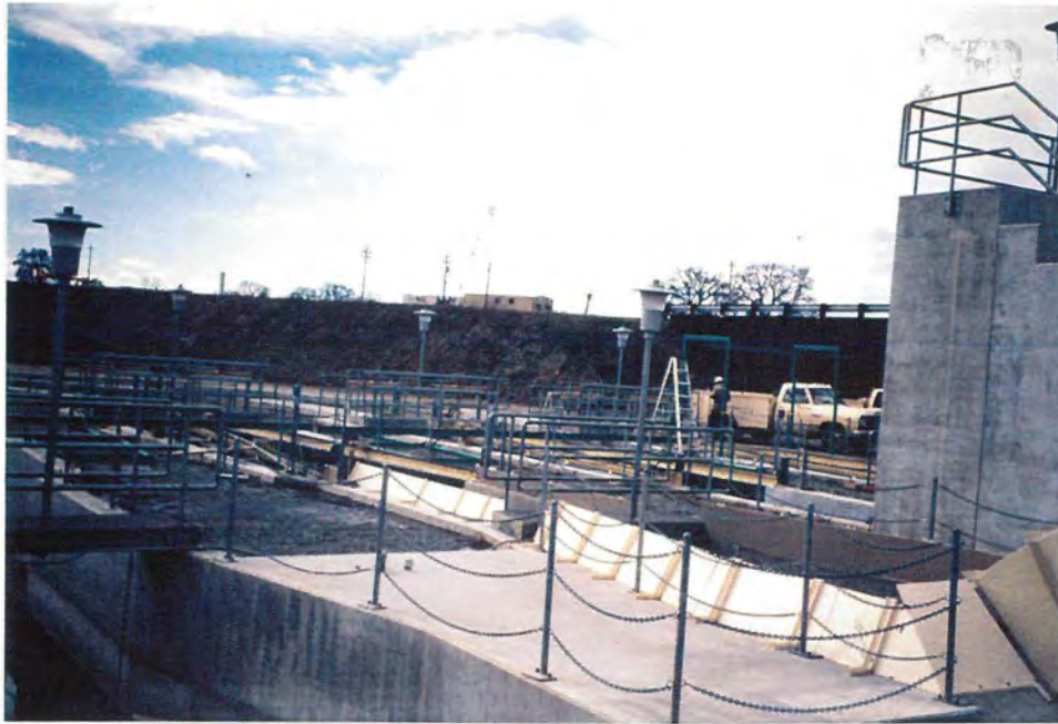
Figure 10: Splashguards installed on bay No. 3.
