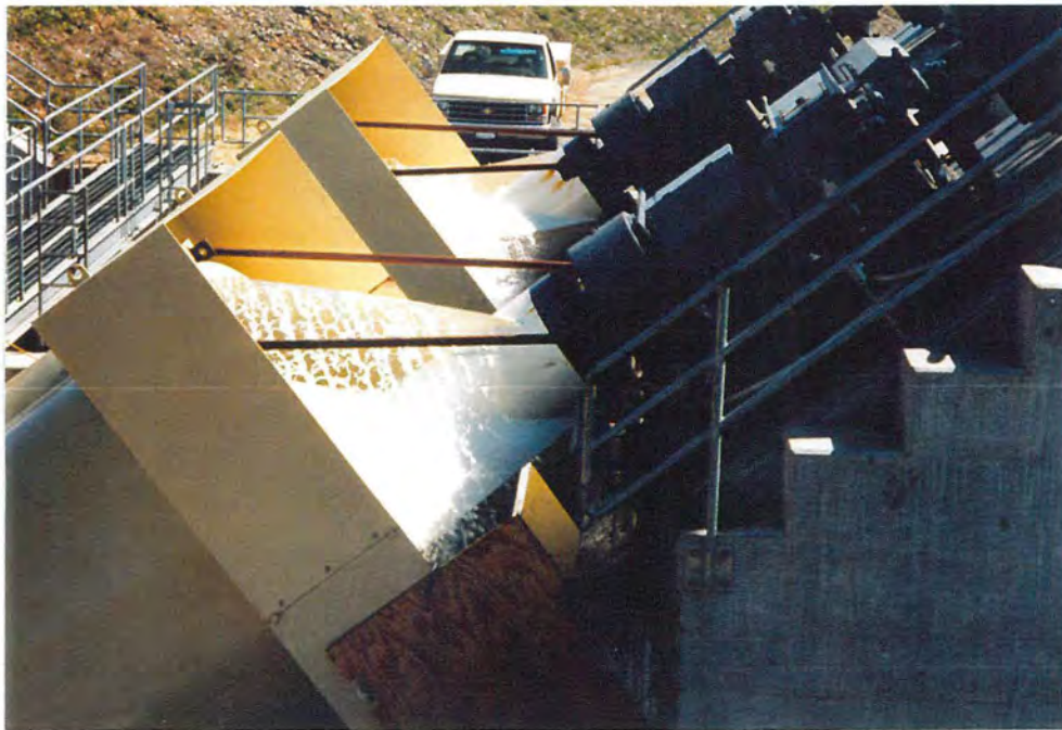
Figure 11: Carryover splashing at the Archimedes pump exit.
