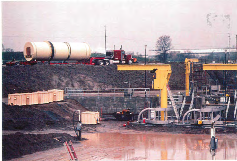
Figure 3: Archimedes pump being delivered to the construction site on a semi-trailer.
