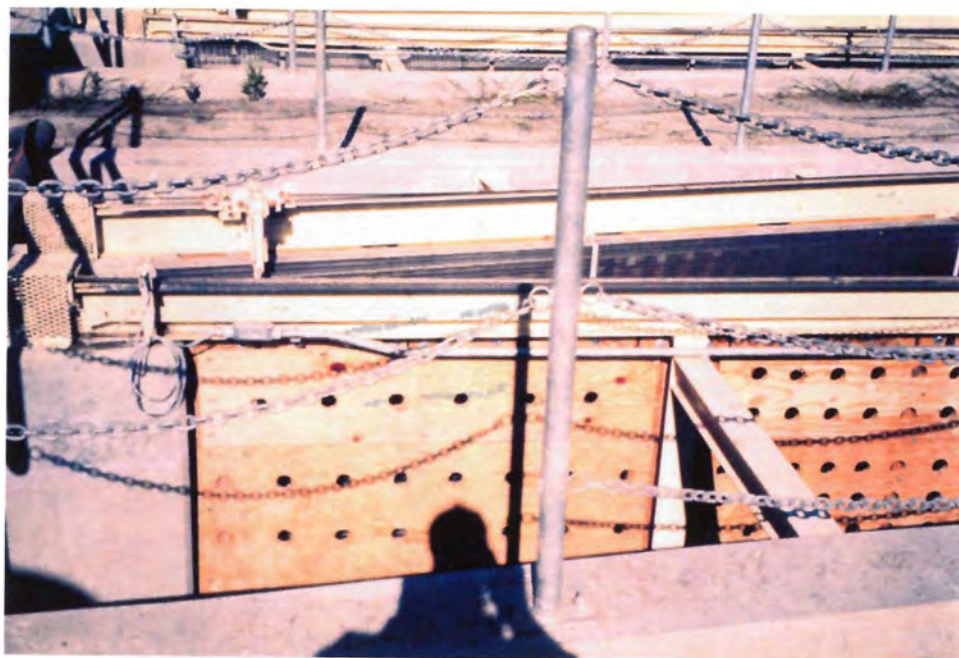
Figure 12: Temporary baffles on the vertical screen structures.
