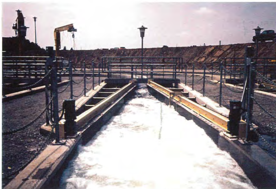
Figure 5: Vertical screen structure and bypass entrance.
