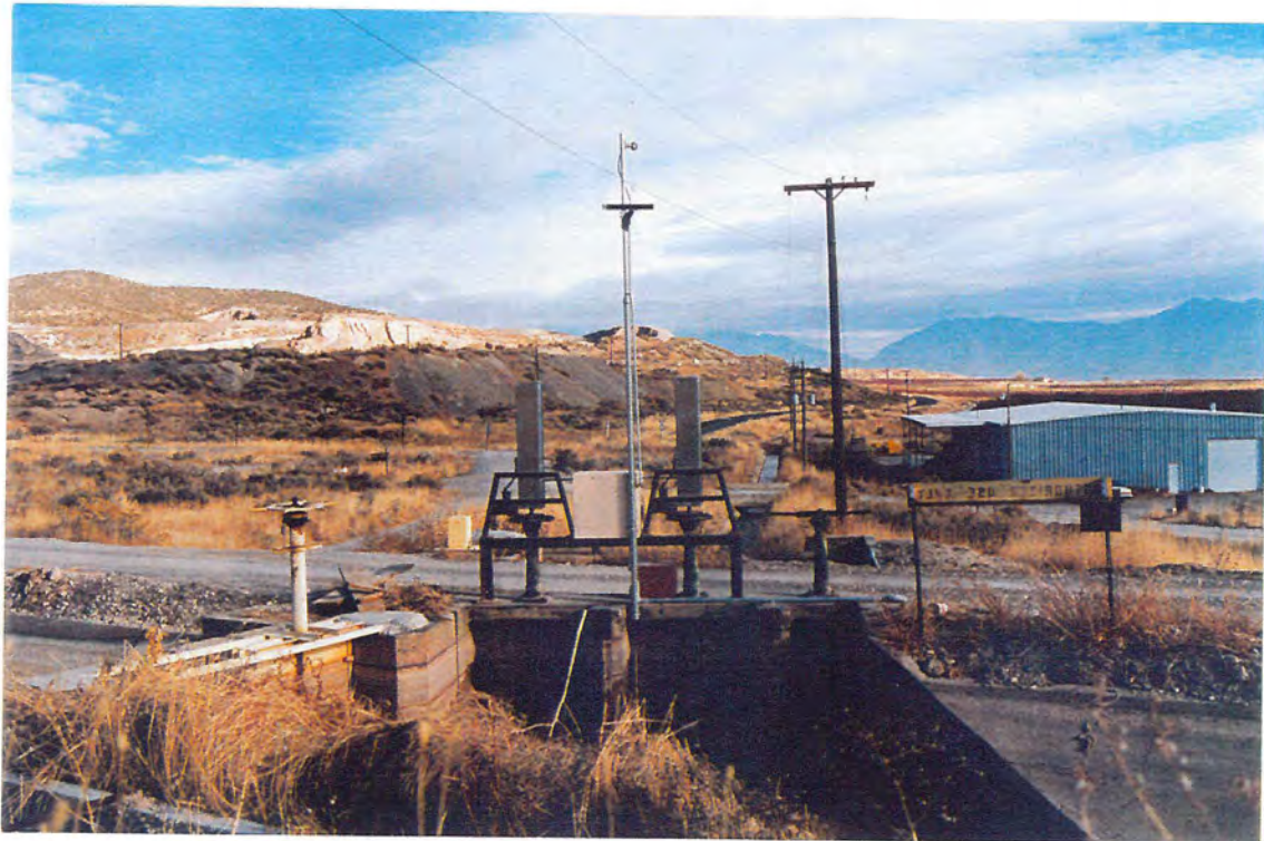
Photograph 4 - Lateral 30, Strawberry High Line Canal, after installation of gate actuators and canal automation equipment (1995).
