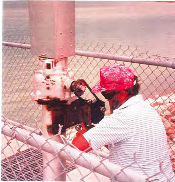
Photograph 5 - Upgrading the real-time system from monitoring to remote control, on Huntington North Reservoir. Emery district staff can now change reservoir releases from their office or mobile unit.
