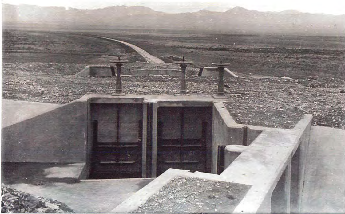
Photograph 3 - Strawberry Highline Canal lateral just after its construction (circa 1920).
