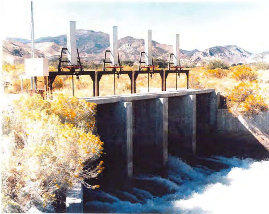
Photograph 3 - Sevier Valley-Piute Diversion after the retrofit of solar-powered automation equipment.
