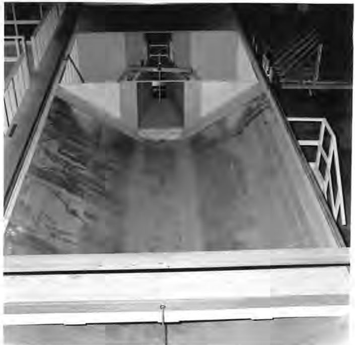
Figure 2. View of "Montana" Parshall flume installation (looking downstream).
