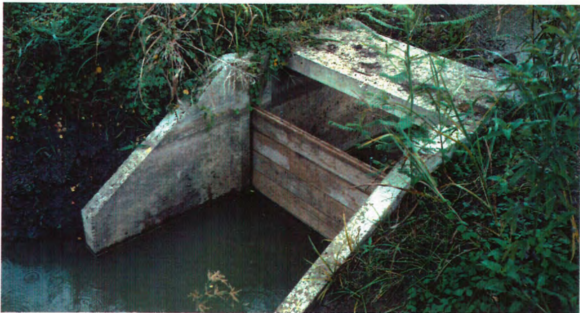
View of a "undershot" farm delivery structure.
