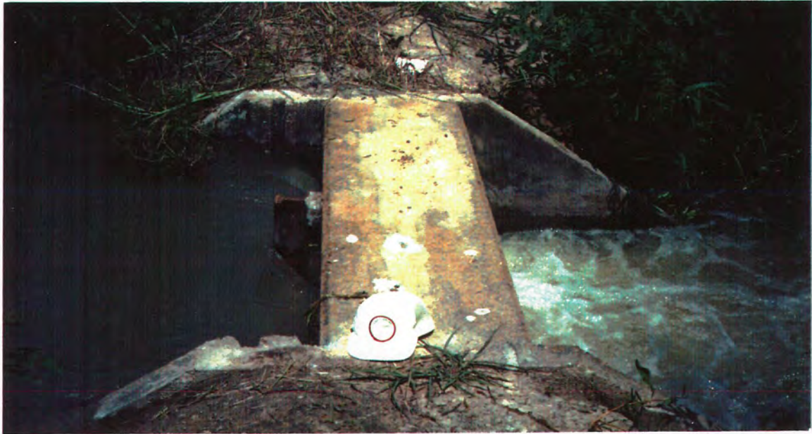
View of a canal "overshot" flow-control device.
