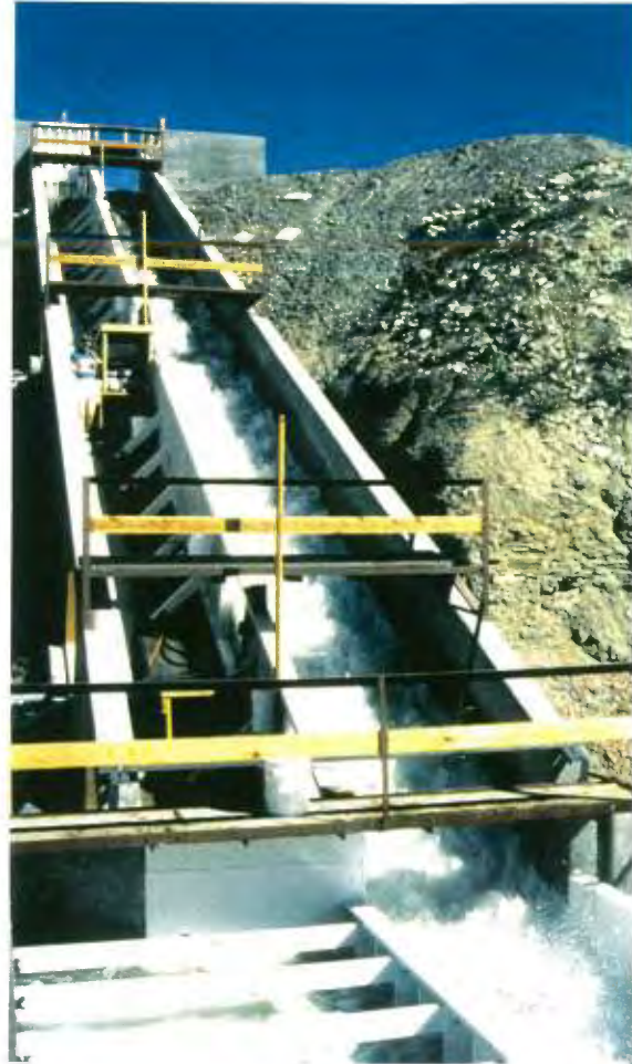
Figure 4B. - View of the 1.5-m-wide, 15-m-high test facility at CSU discharging 3.0 \text{ m}^3/\text{s} .
