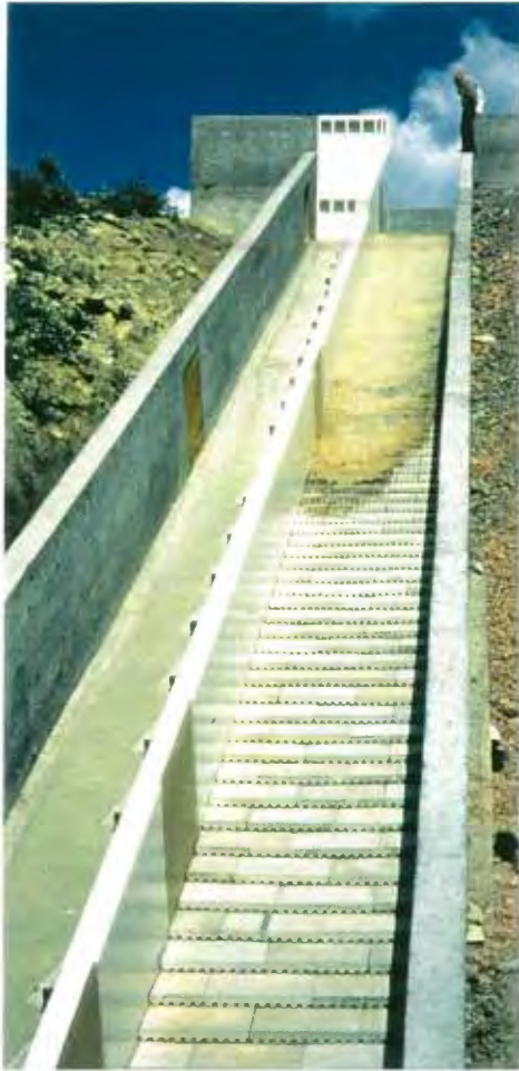
Figure 4A. - View of flow starting over the 2:1 slope. Blocks are placed in an overlapping fashion on 15 cm of gravel.
