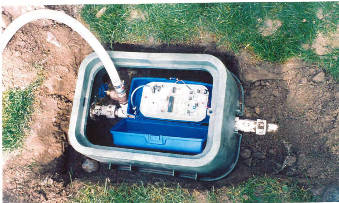
Figure 12. Completed installation showing hose for field calibration test.
