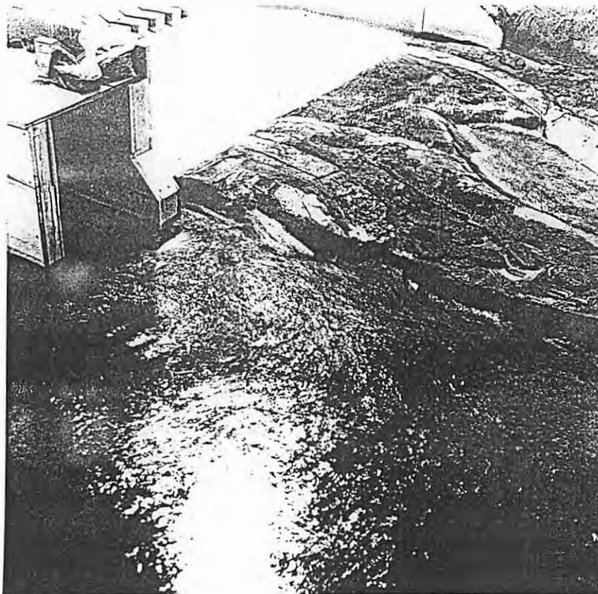
Figure 13. - Channel B with only the far left gate operating at 8,000 ft 3 /s with no powerplant flow.
