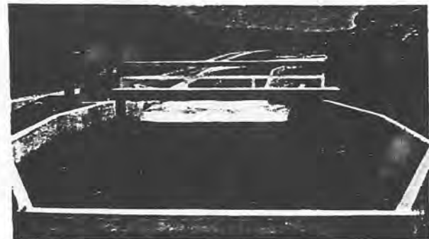
Figure 12. Underpass-type wave suppressor significantly reduces turbulence and waves in Parshall flume, making accurate discharge determination a routine matter. Photo P245-D-30663
