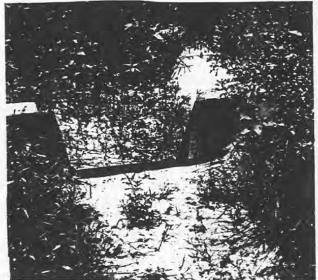
Figure 14. Sediment deposits have reduced the depth of the weir pool sufficiently to increase the velocity of approach to well above the desirable level. The head gage should not be located close to the weir blade. The weeds should be removed and the "edge" of the weir should be sharp. Discharges over this weir will be larger than indicated in "standard" tables. Photo P20-D-21558
