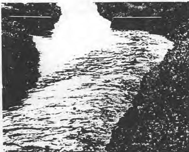
Figure 8. Poor approach flow conditions upstream from weir. The high-velocity, turbulent stream is approaching the weir at a considerable angle. Head measurement is difficult, and the weir does not discharge a "standard" quantity. Photo PX-D-30664
