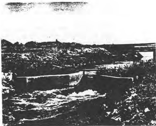
Figure 28. Four-foot Parshall flume discharging 62 cfs under free-flow conditions. Downstream scour protection is required with this height of fall. Photo PX-D-55348
