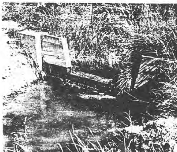
Figure 17. Weeds protruding through the opening and sediment in the approach pool will result in inaccurate discharge determinations. Photo P-D-30665
