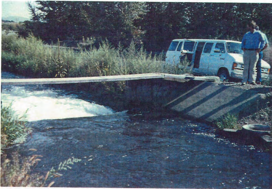
Photo No 4- Rated drop in Track Lateral that could be replaced with a weir.
