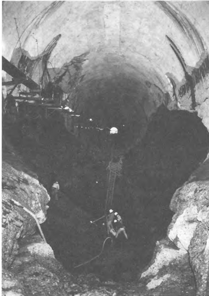
Figure 8. - View looking downstream across the 10.7-m-deep hole in the invert liner of the left tunnel spillway at Glen Canyon Dam (Burgi and Eckley 1987).
