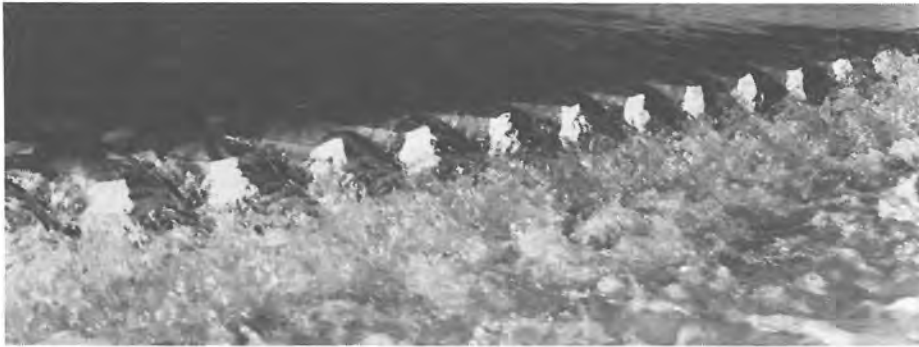
Figure 4. - Ute Dam labyrinth spillway with 15 575 m 3 /s (Houston 1982)
