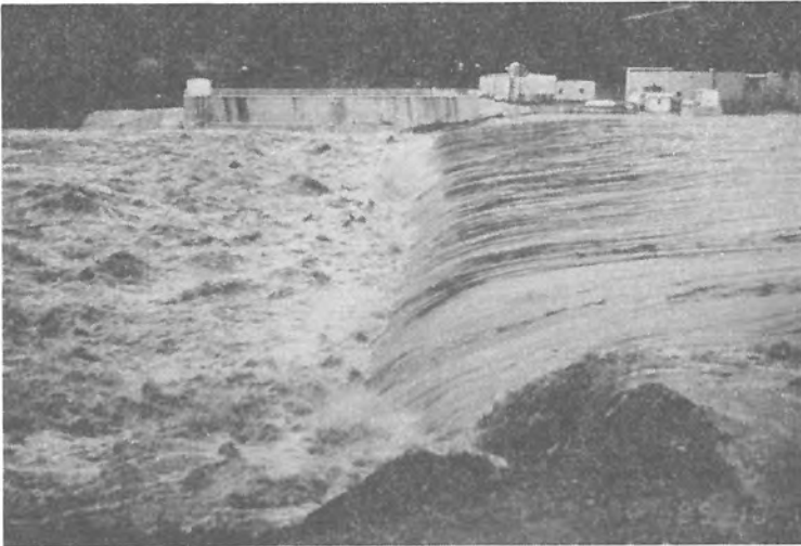
Figure 9a. - Kirville Dam - 4.3-m overtopping.
