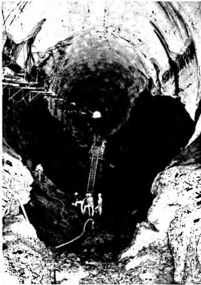
Figure 4. View looking downstream across the 10.7-m-deep hole in the invert liner at base of the vertical bend - left tunnel spillway. September 1983.
