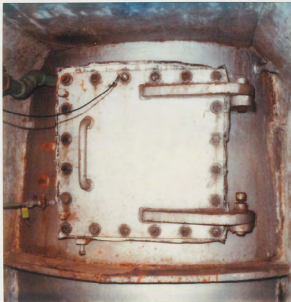
Fig-3. Accelerometer location on Mandoor of Draft Tubes of Flatiron Units 1 and 2
