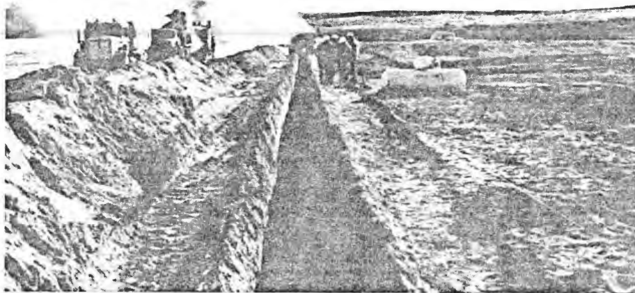
Figure 1-12. - Excavation of key trench.
