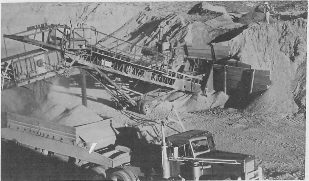
FIGURE 18. - View of earth-moving and screening equipment operations in the borrow pit.
