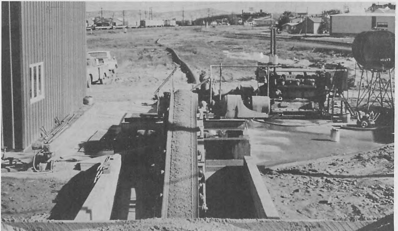
FIGURE 19. - View of end of hopper, conveyor, slurry pump, diesel engine, pipelines and control building at mixing plant.
