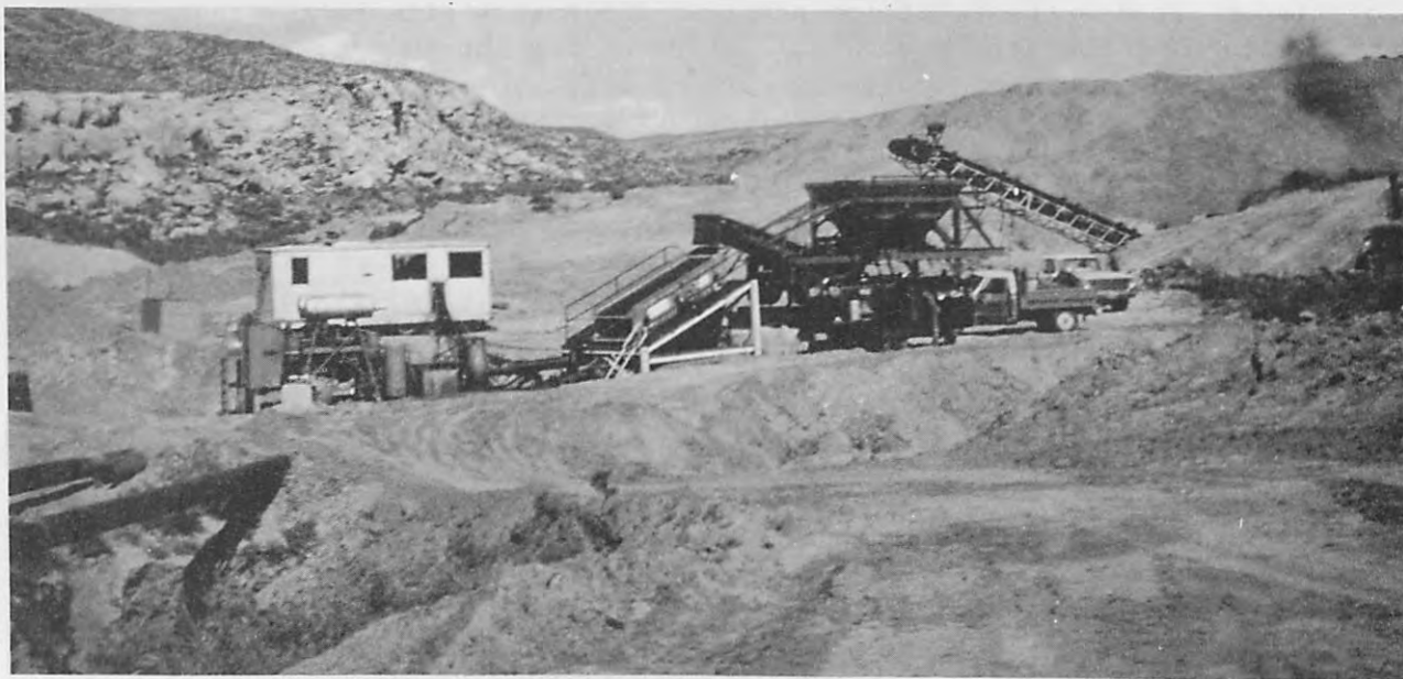
FIGURE 14. - View of the slurry mixing plant installation at the site of the borrow pit about 2 miles from the built-up areas of the city. Note natural rock outcropping in left background off project limits and slurry pipeline in left foreground.
