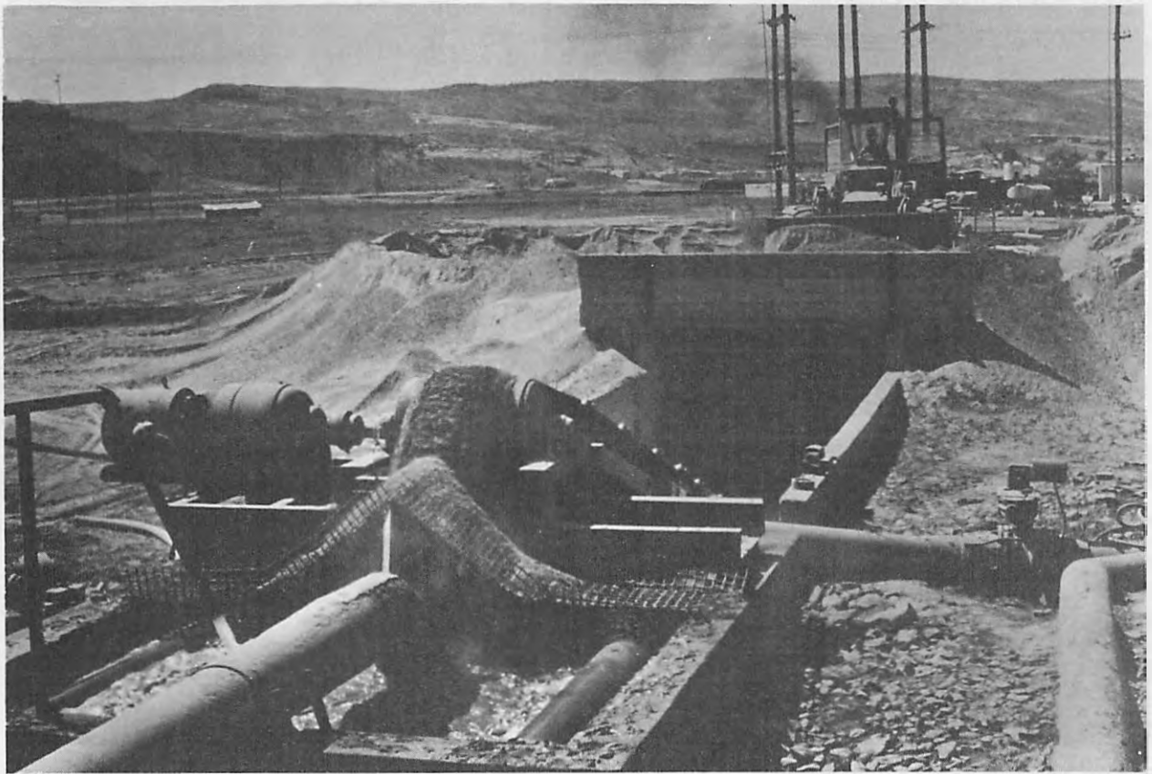
FIGURE 20. - View of mixing tank, suction line, sand being delivered to mixing tank, and bulldozer in the background pushing sand into hopper.
