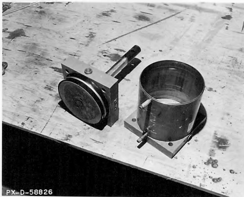
a. General View of The Parts of Hydraulic Cylinder
