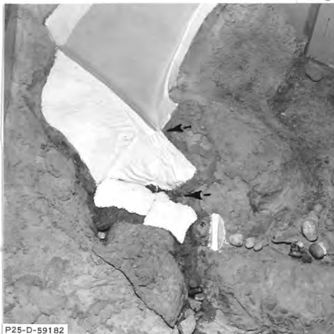
A. Recommended additional concrete paving is indicated by the arrows
