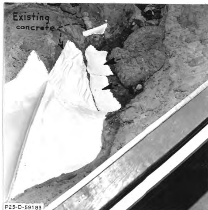
B. Recommended additional concrete fill is indicated by the arrows
